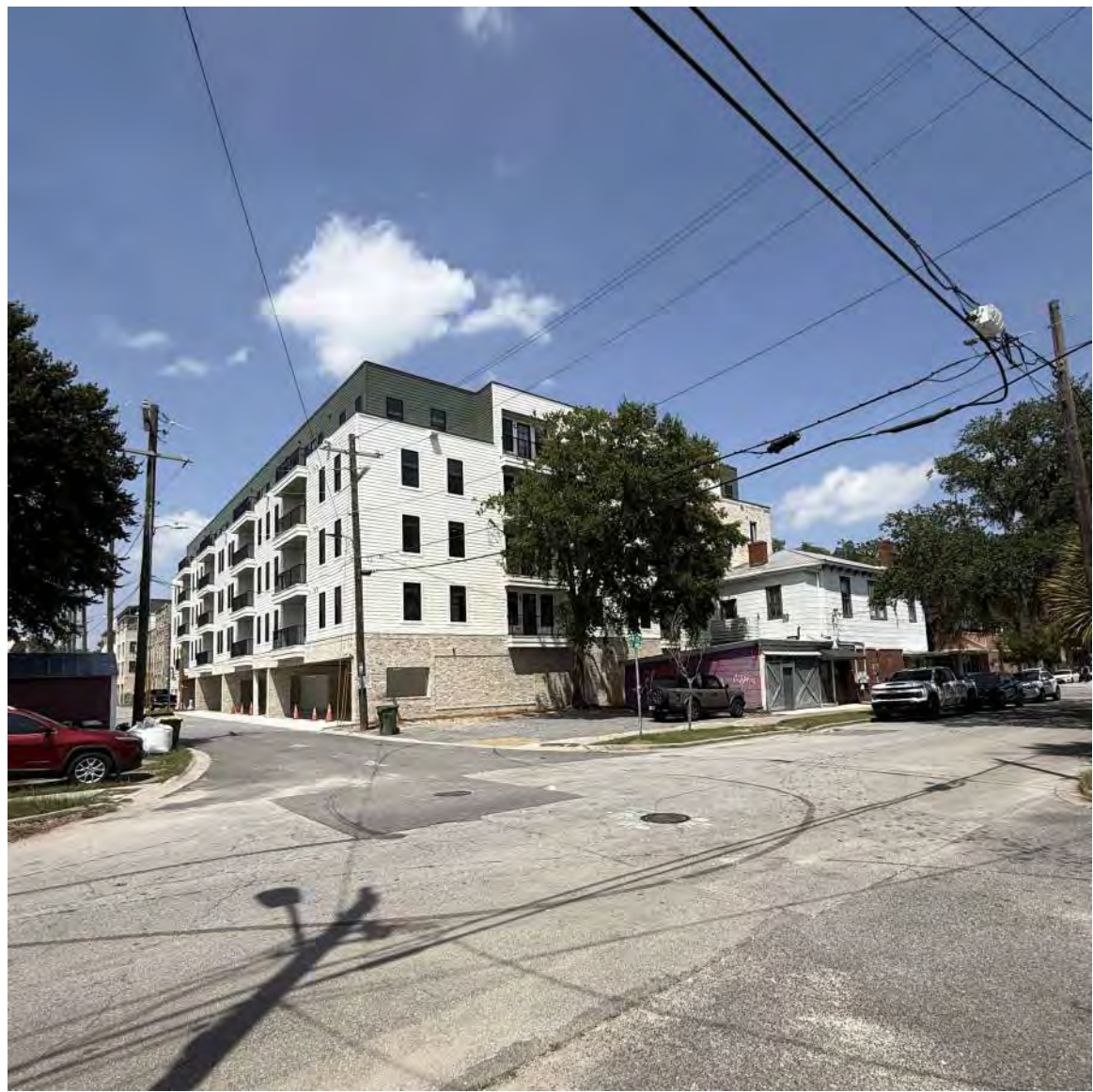
DESOTO AVE- FACING NORTHEAST
