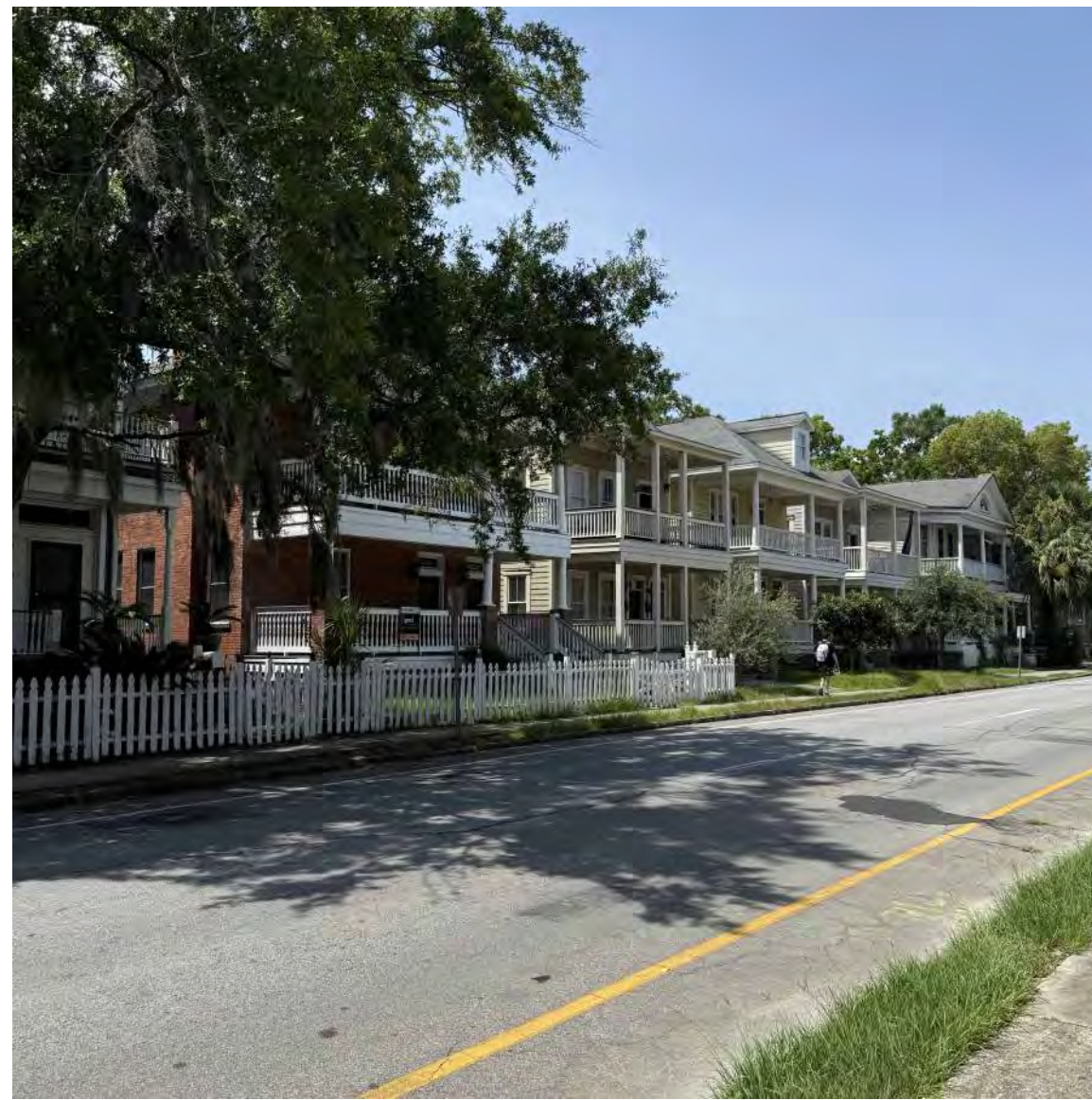
WHITAKER STREET- FACING NORTHWEST
