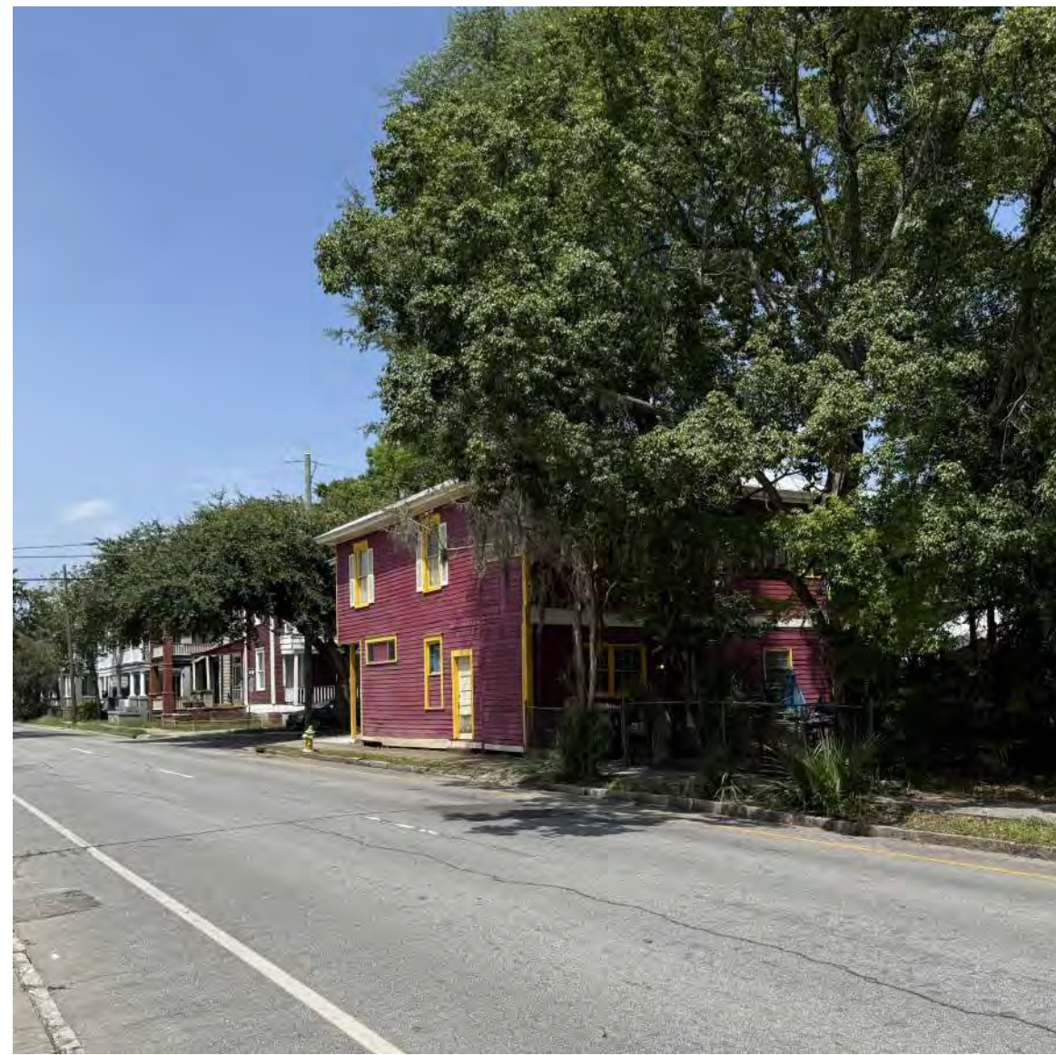
WHITAKER STREET- FACING NORTHEAST
