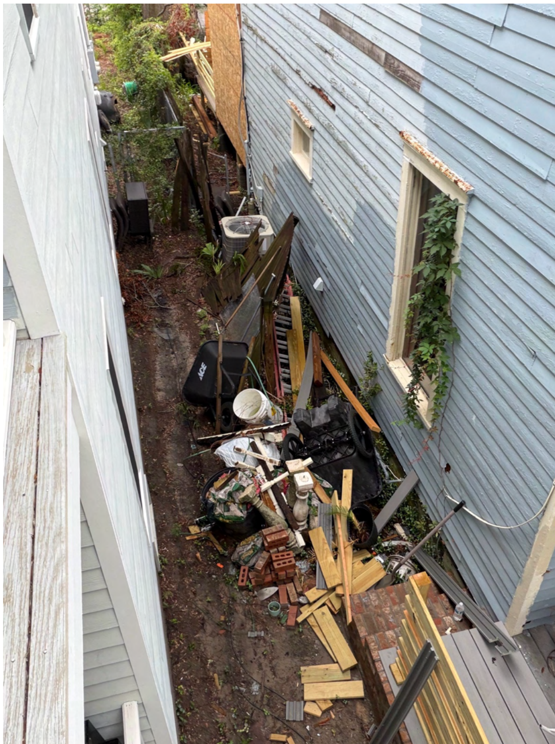
My house is on the left side; neighbor's house is on the right side. Dilapidated wood fence in between the neighbors overflowing trash to be replaced.
