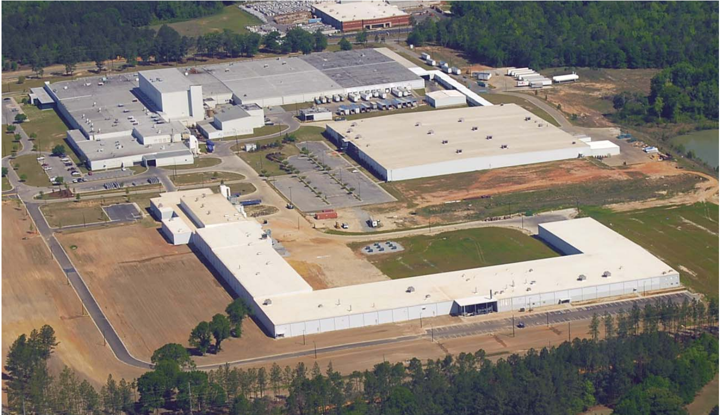
YKK AP maintains a state-of-the-art ISO 14001 certified manufacturing facility in Dublin, Georgia.
