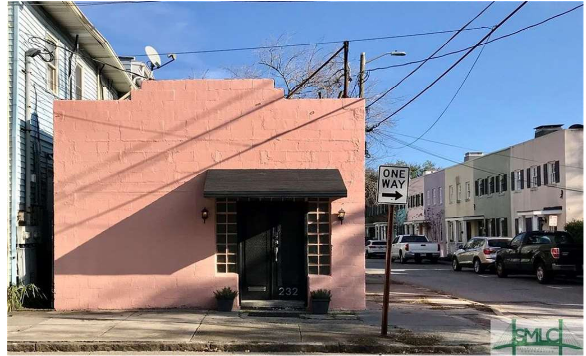
VIEW OF FRONT FACADE
