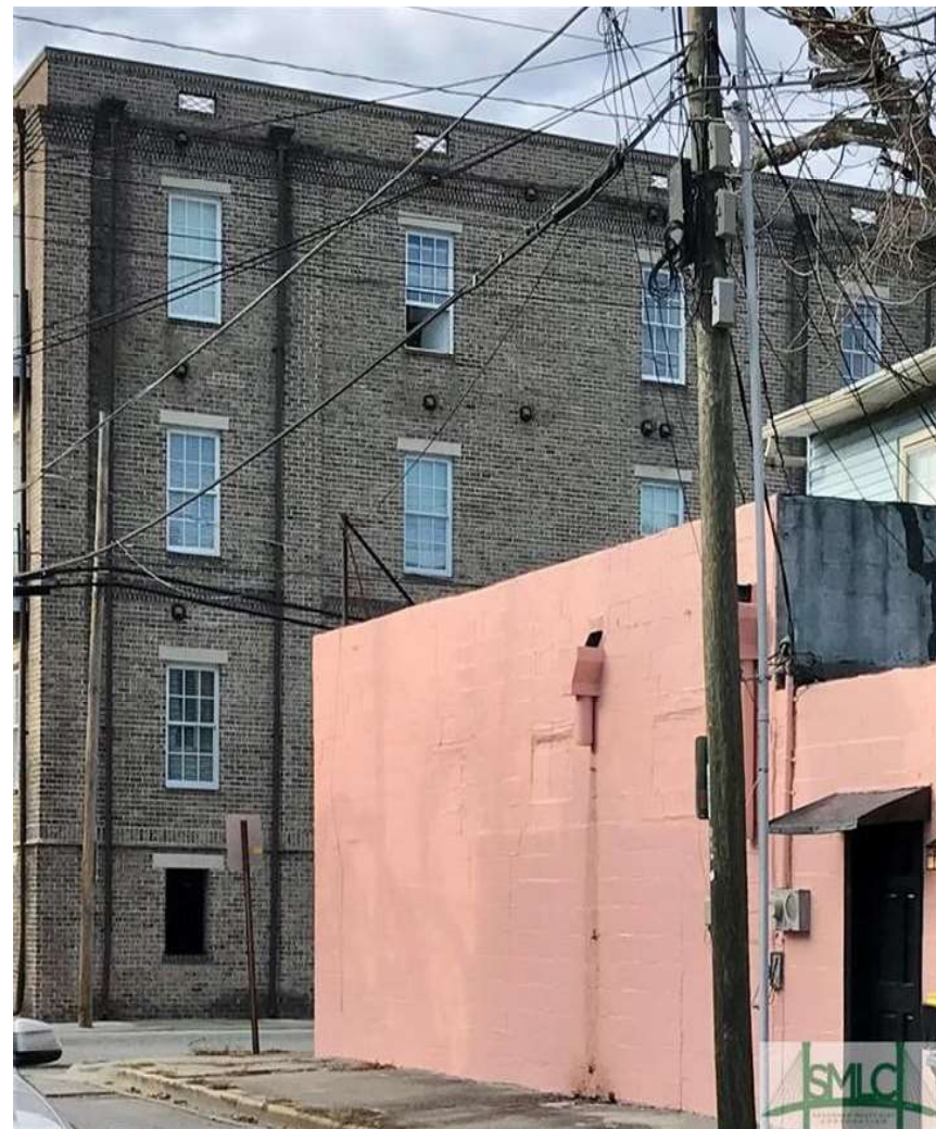
VIEW FROM PERRY ST LOOKING NW
