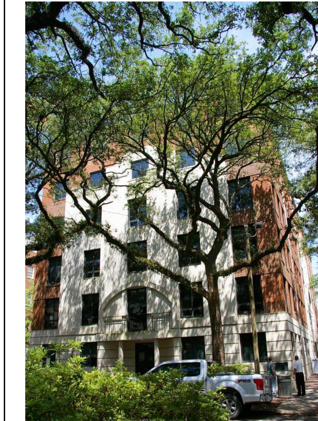
7 HD BR 0.2 EXISTING SITE CONTEXT PHOTOS - 200 E. ST. JULIAN N.T.S.
