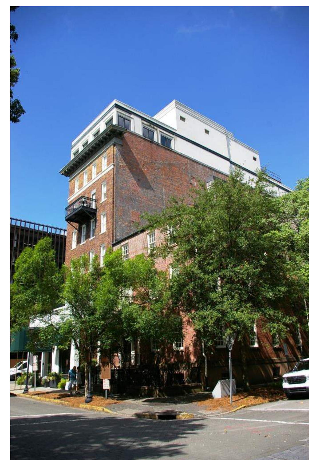
8 HD BR 0.2 EXISTING SITE CONTEXT PHOTOS - 29 ABERCORN STREET N.T.S.
