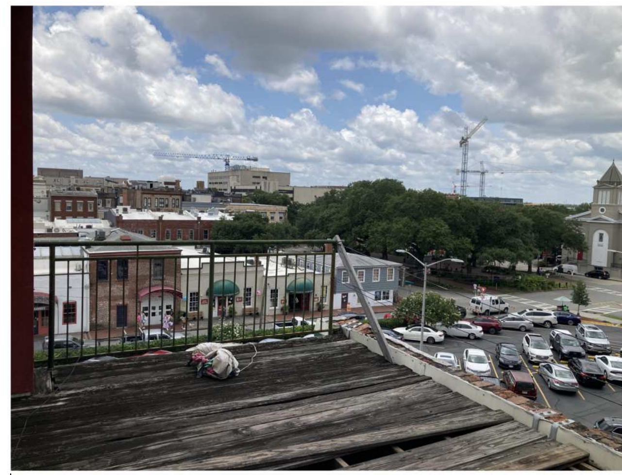
REFER TO KEY NOTES 6 8 & 9 REPLACE DAMAGED EXISTING DECK
