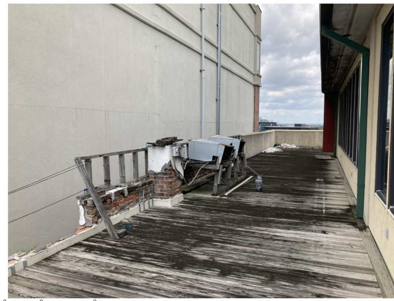
REFER TO KEY NOTES 6 8 & 9 REPLACE DAMAGED EXISTING DECK
