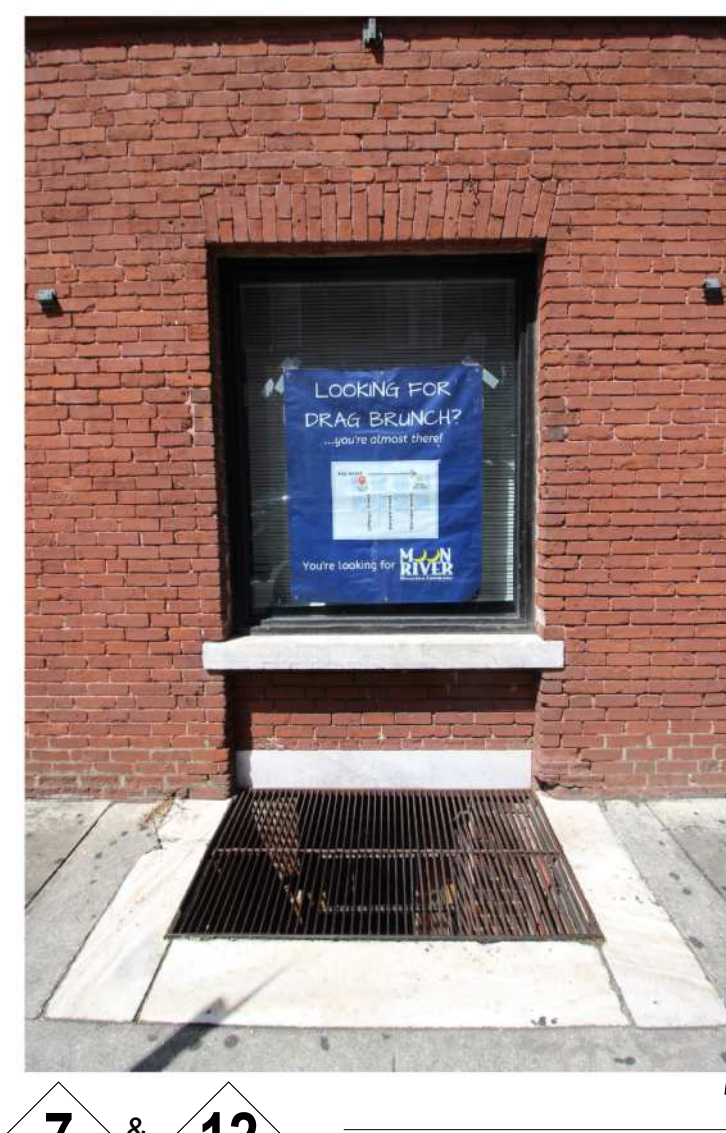
REFER TO KEY NOTES 7 & 12 REPLACE EXISTING SIDEWALK GRATING
