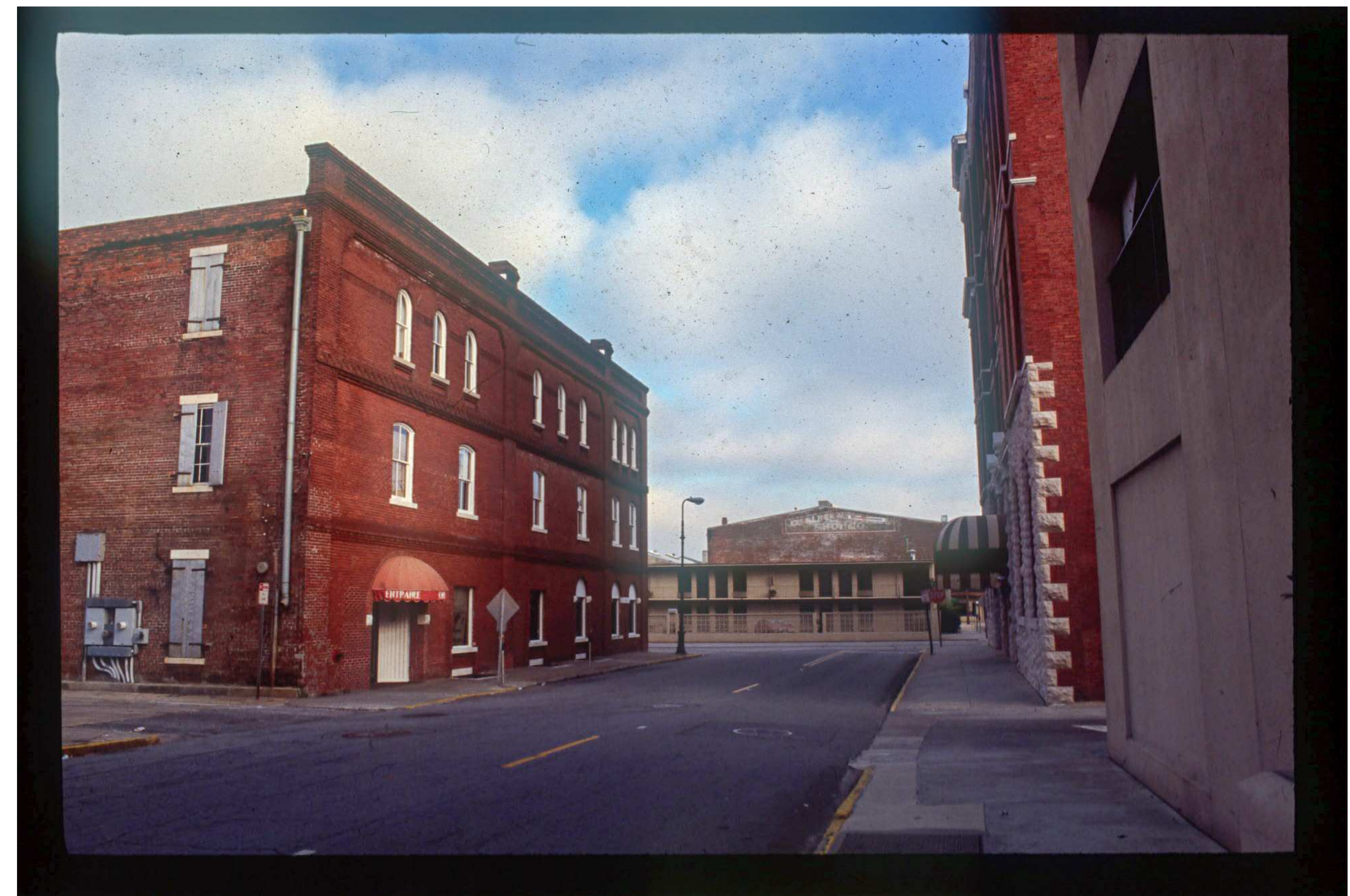
NORTH FACING VIEW FROM JEFFERSON STREET - CIRCA 1980s
