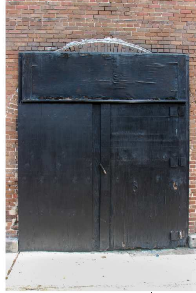
REFER TO KEY NOTE 1 REPAIR BRICK @ BASE OF OPENING
