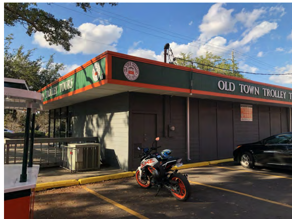
SOUTH EAST CORNER
