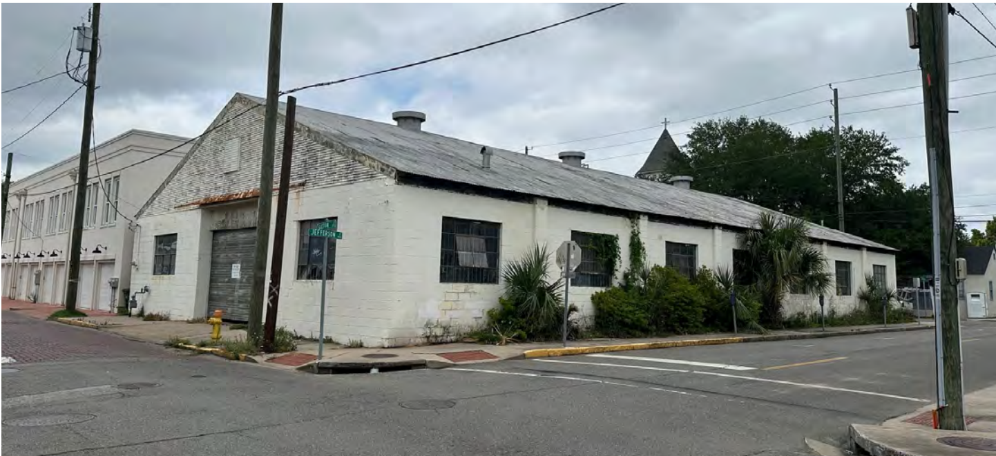
View looking north west.
