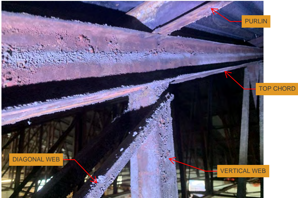
Photo 8: Roof truss – Web and Top Chord Connections
