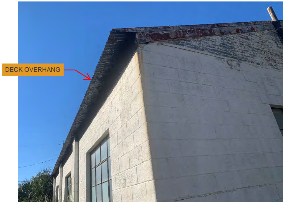
Photo 3: Roof decking – Cantilevered eave
