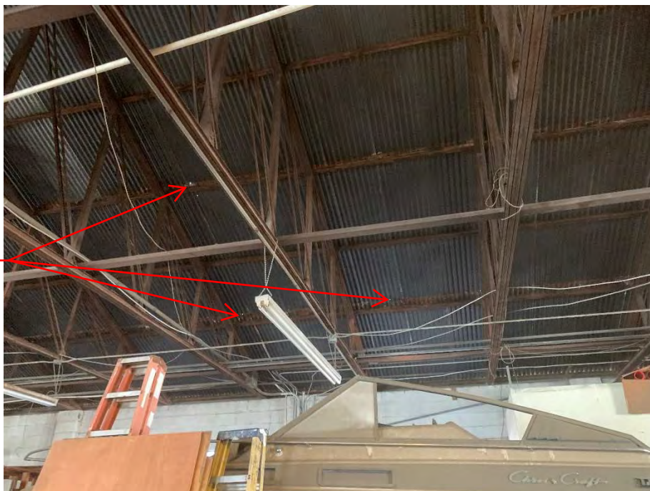
Photo 2: Roof decking - Holes in decking
