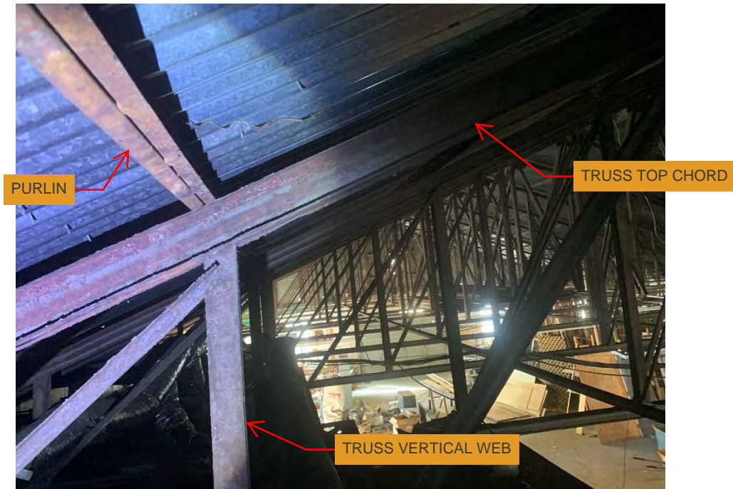
Photo 4: Purlins – Light-gauge and shallow member
