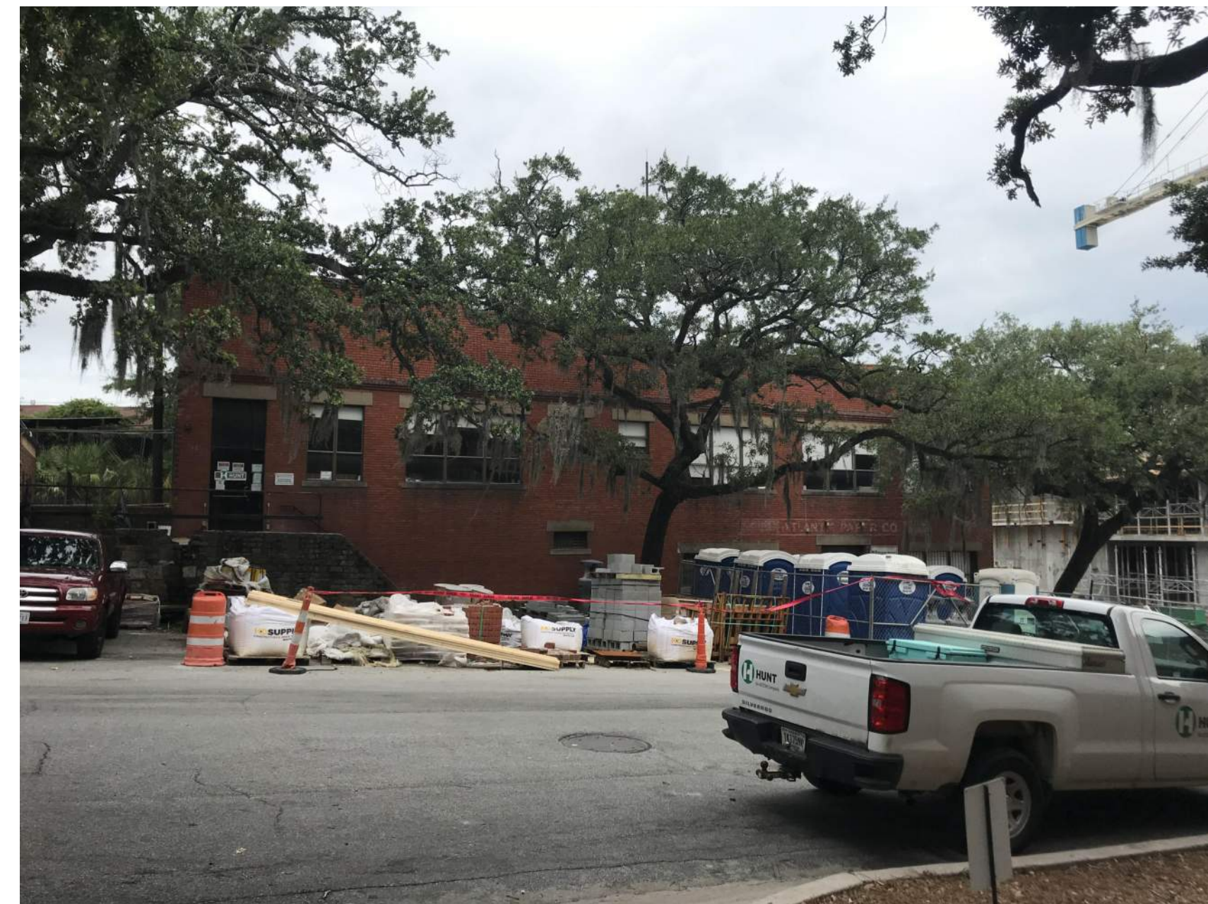
VIEW FROM MARTIN LUTHER KING JR. BLVD.
