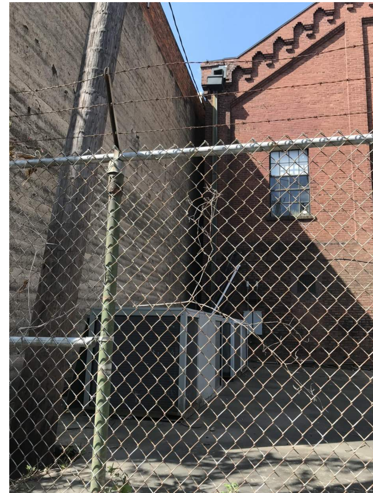
VIEW FROM RIVER STREET OF ADJACENT BUILDING TO WEST
