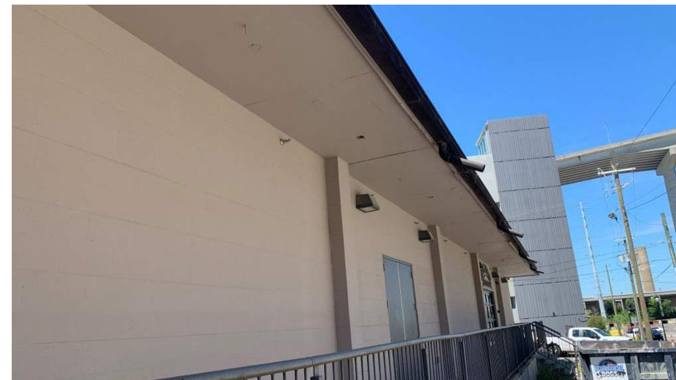
NORTH ELEVATION VIEWING WEST
