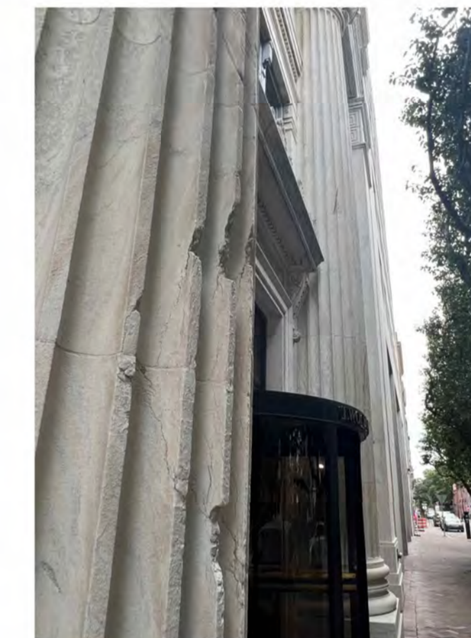
06- EXISTING MARBLE COLUMN TO BE REPAIR
