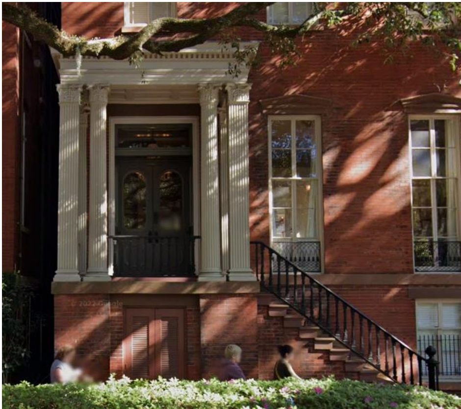
10 West Jones Street - brick, wood, and iron design.
