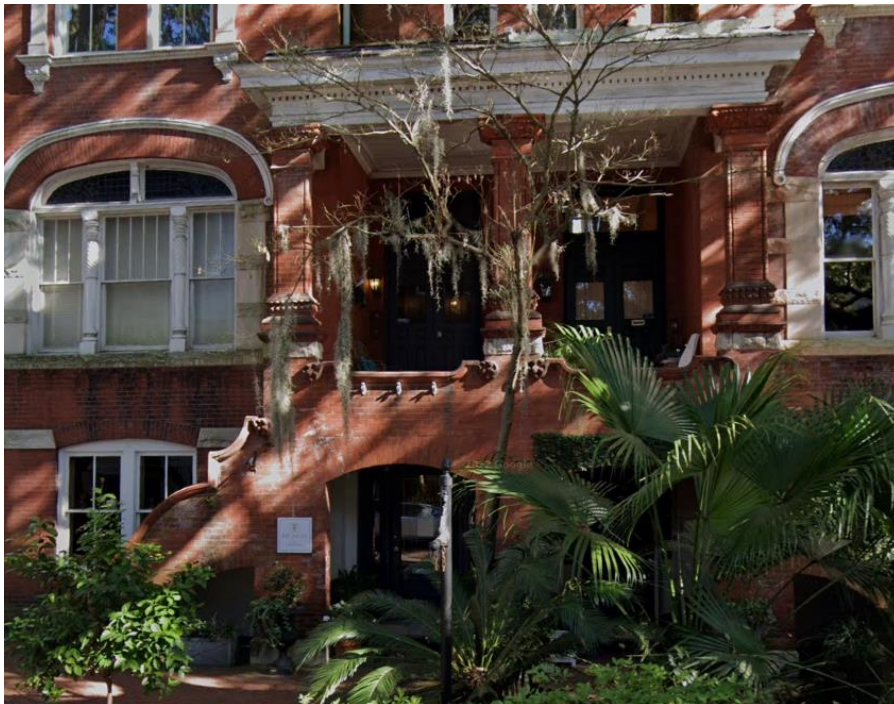
12-14 West Jones - brick, terra cotta, and wood design.
