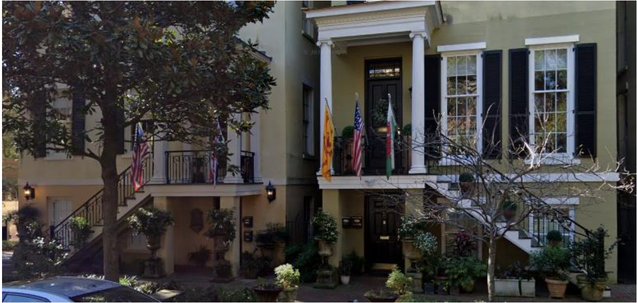
1-3 West Jones Street - wood, stucco, and iron design.
