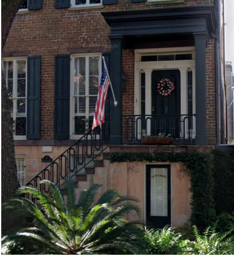
11 West Jones Street - stucco, wood, and iron design.
