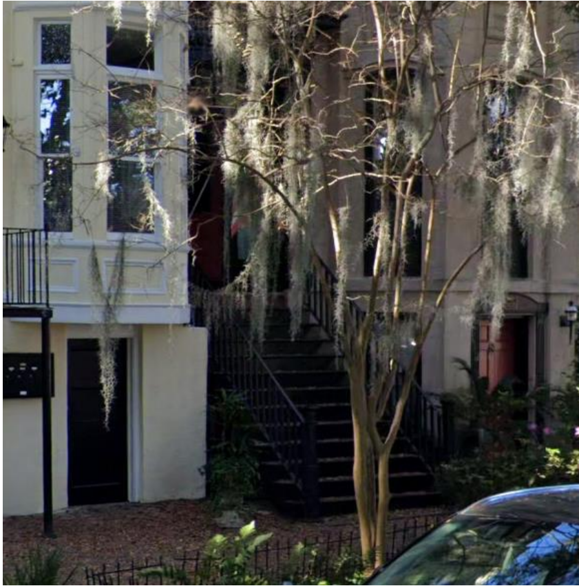
17 West Jones Street - New stoop.
