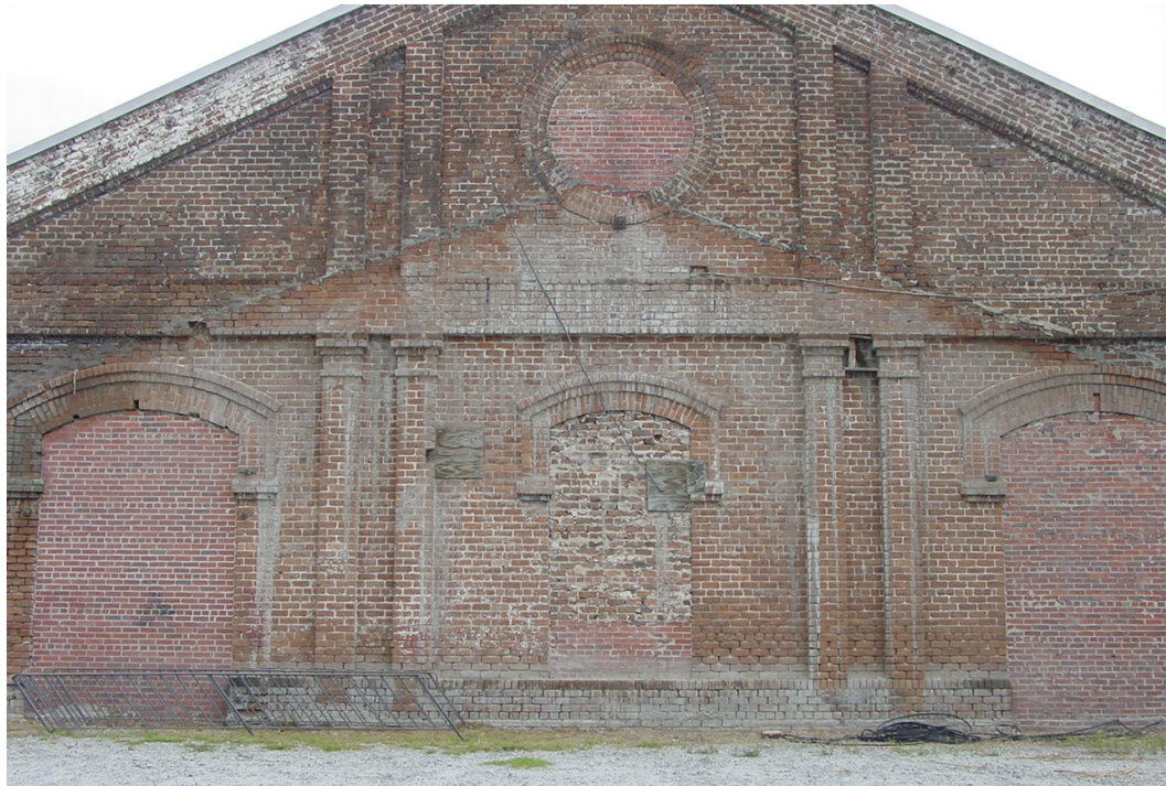
South façade of Morris Center before and after paint removal
