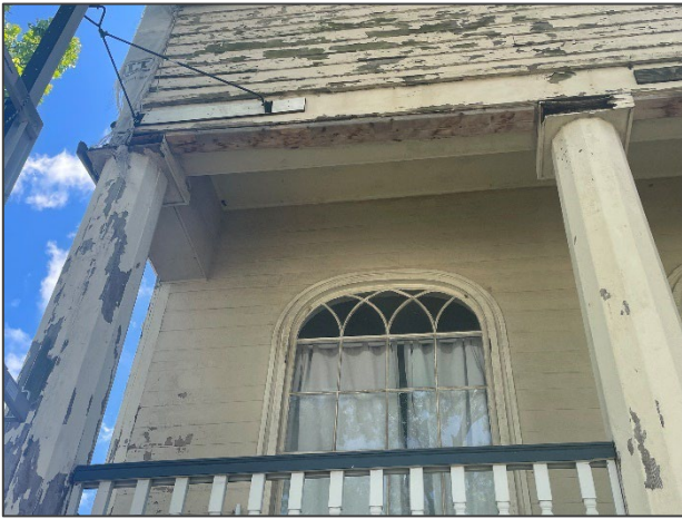
Current site photos taken by MPC staff
