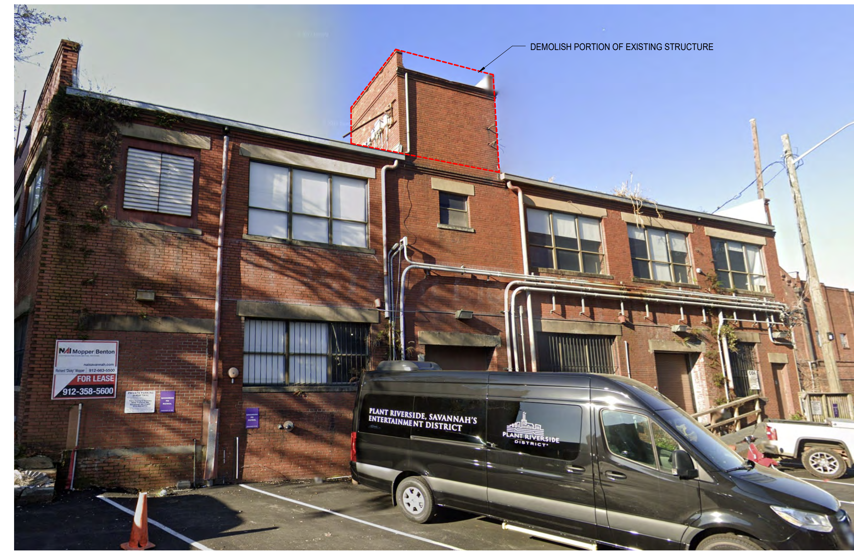
DEMOLITION ELEVATION (RIVER ST)
