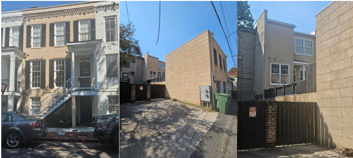
Staff Site Visit Photos – Confirmation of Posting; views of front (West Taylor Street) and rear (West Jones Lane) elevations
