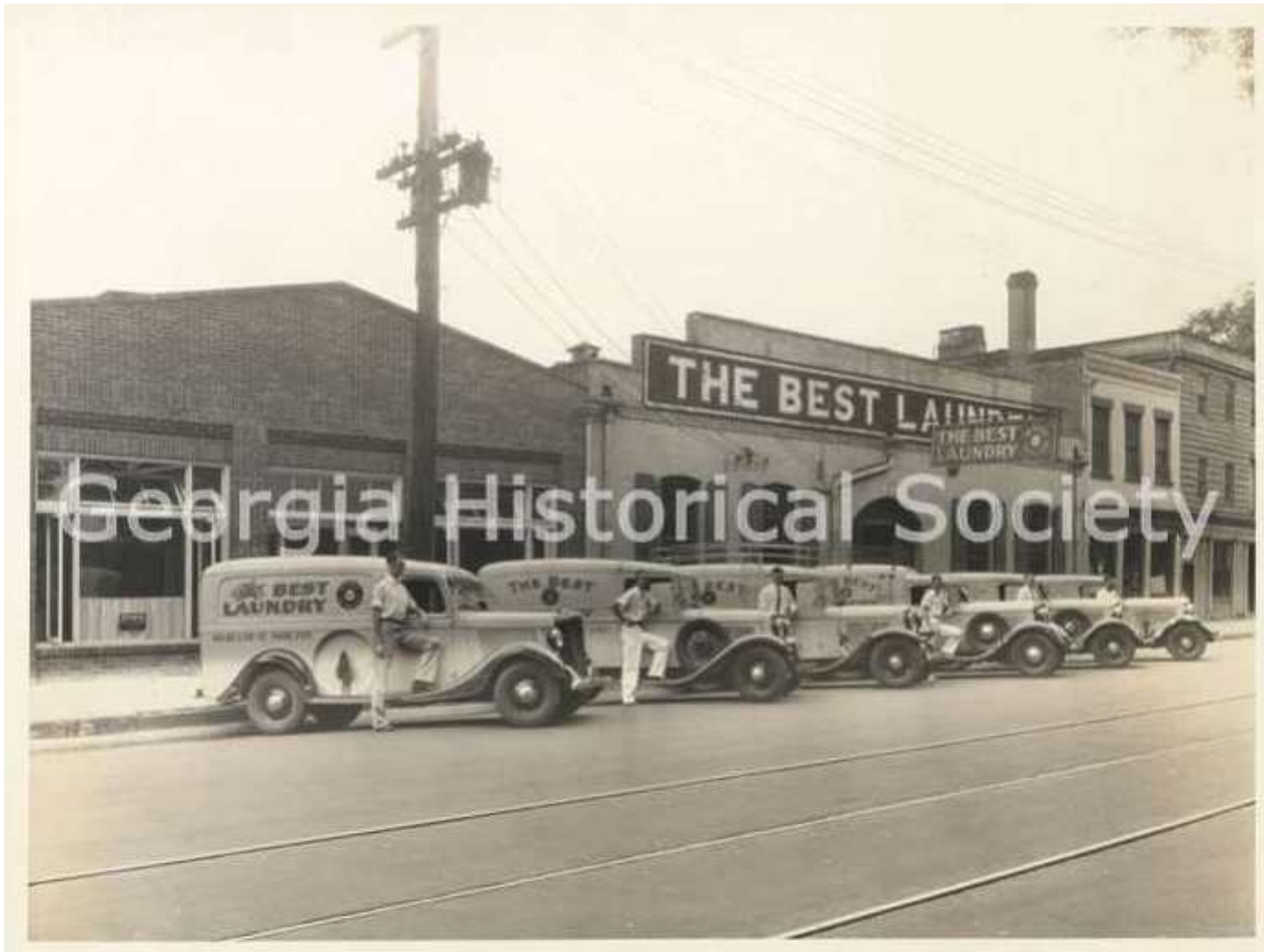
HISTORIC BAY STREET
