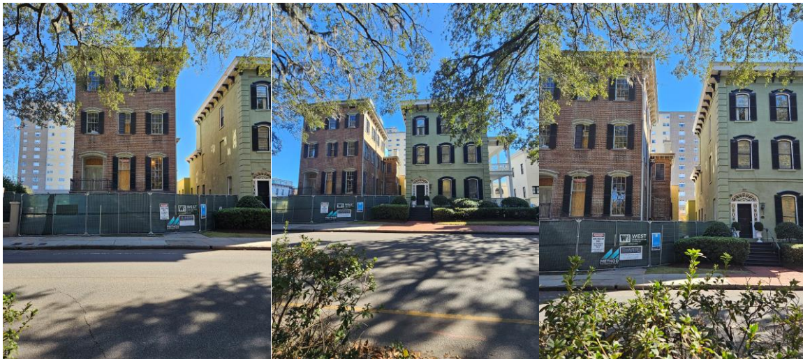
Staff Site Visit Photos – Views of front elevations of both 612 & 618 Drayton Street
