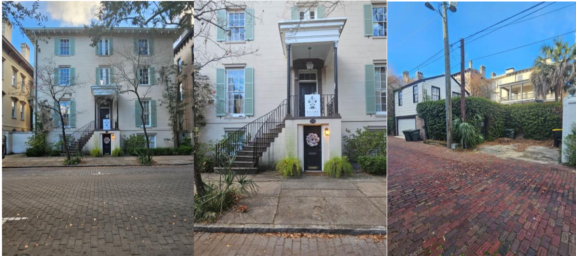
Staff Site Visit Photos – views of front (West Gordon Street) elevation and rear (West Gordon Lane) elevation
