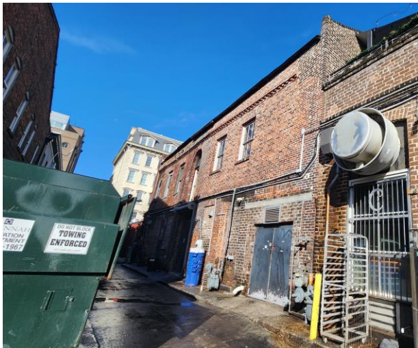
Figure 10. Rear of the Accessory Building.
