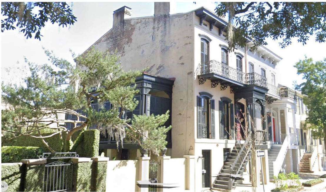
CONNECTED ROW HOUSE SLEEPING PORCH ON SIDE
