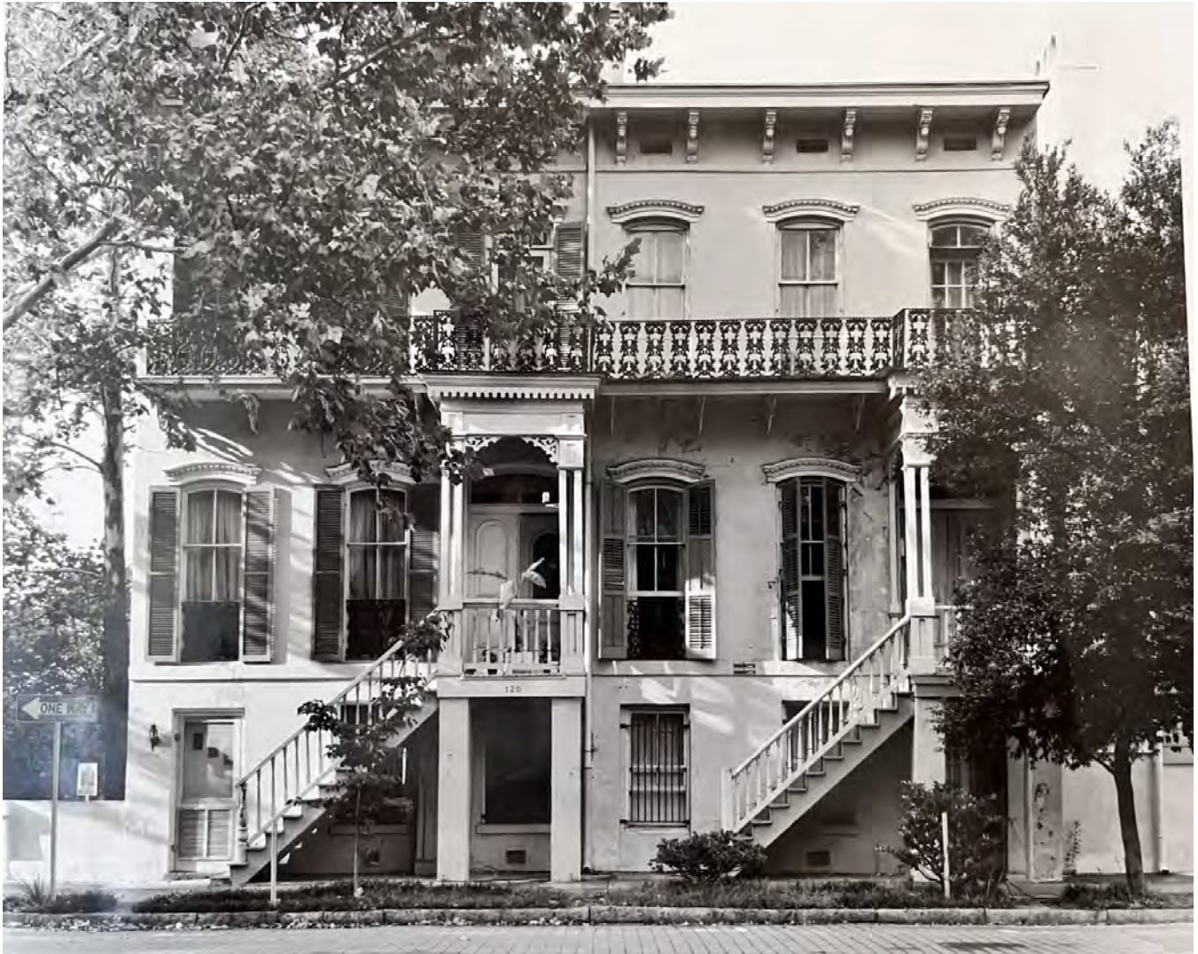
118-120 West Harris Street, undated. Historic Savannah Foundation.
