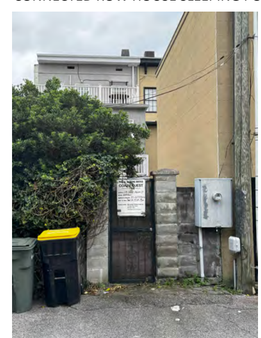
EXISTING SPACE BETWEEN EXISTING ADDITION AND CONNECTED ROW HOUSE CARRIAGE HOUSE
