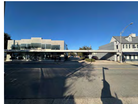
402 BROUGHTON- EXISTING CONDITIONS
