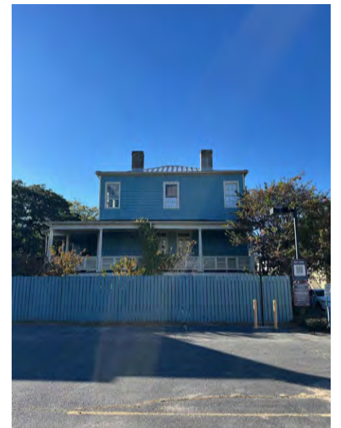
401 E. BROUGHTON ST - looking west
