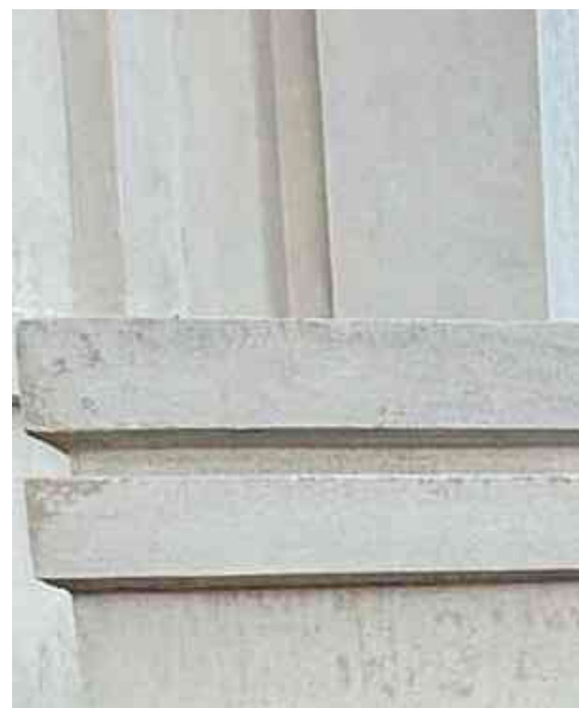
EXISTING STUCCO WALL
