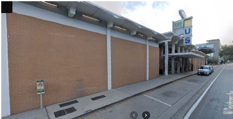
1. Contributing Greyhound bus station built in 1965
