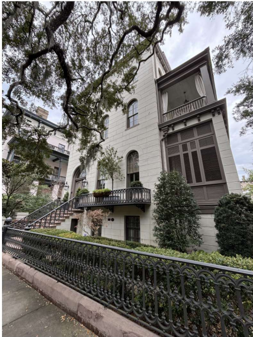
VIEW OF HOUSE FROM W. GASTON
