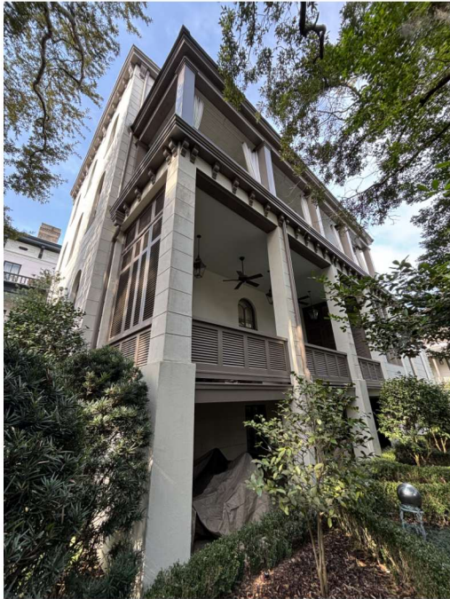
EAST ELEVATION OF SIDE PORCHES
