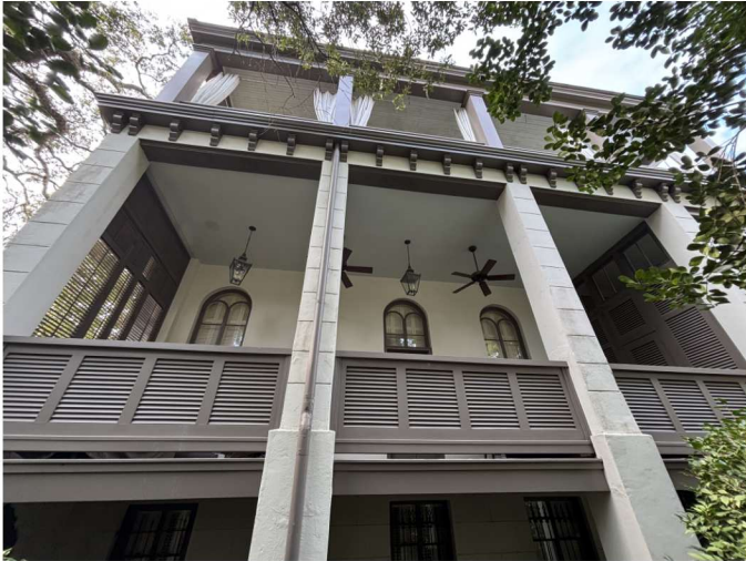
EAST ELEVATION OF SIDE PORCHES
