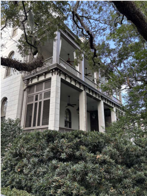
VIEW OF HOUSE FROM W. GASTON
