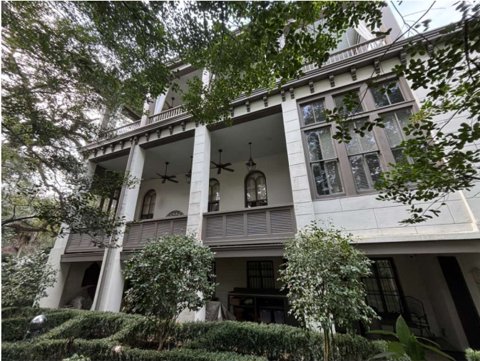
EAST ELEVATION OF SIDE PORCHES
