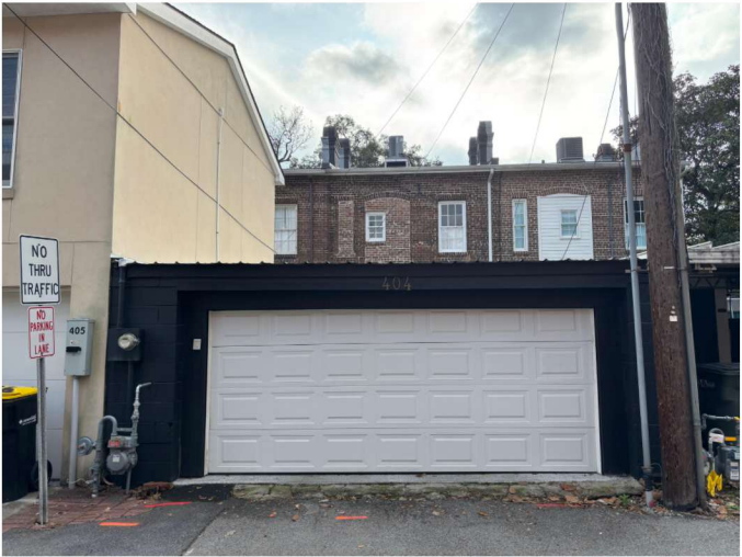
VIEW OF PROPERTY ALONG LANE
