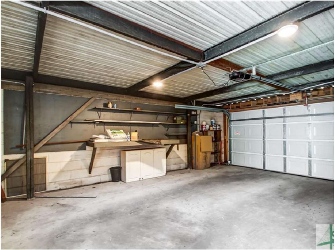
VIEW INSIDE EXISTING GARAGE
