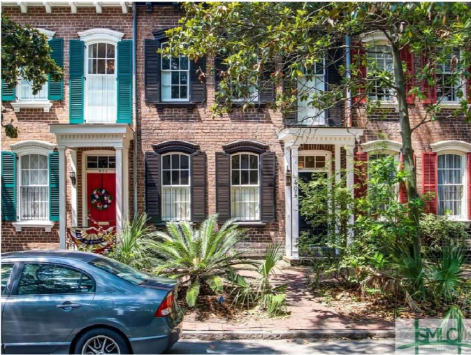
SOUTH FACADE OF TOWNHOUSE
