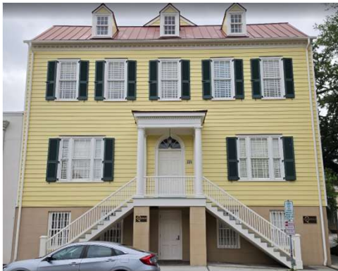
Nearby Structure (1791 Major John Berrien House)
