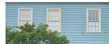
(across Broughton Street, side view)
