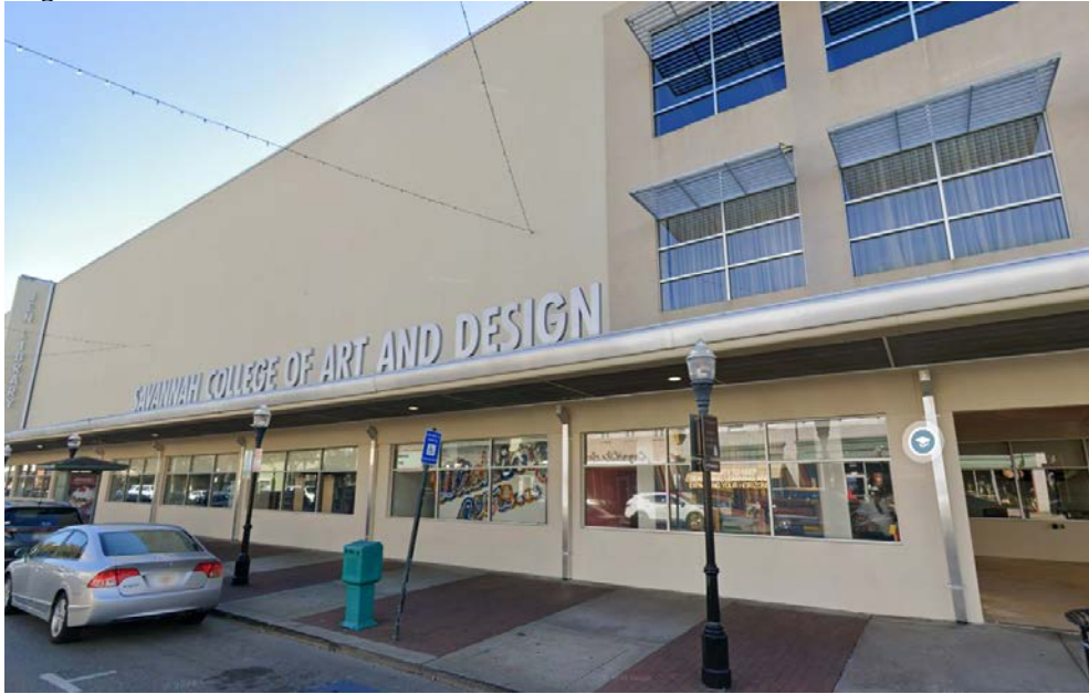
7. 201 East Broughton three blocks east of the subject property – Contributing
