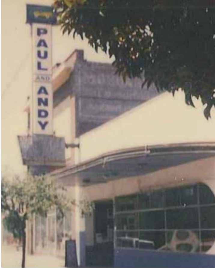
3. Also from 1998 showing the boarded or non-existent second floor windows
