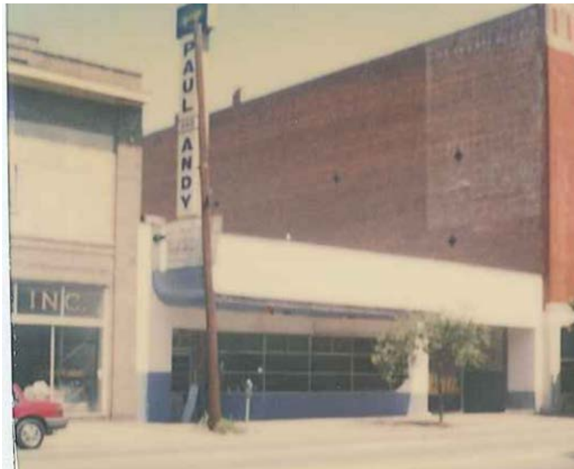
2. Image from 1998 with subject building to the left showing double hung windows either non-existent or boarded
