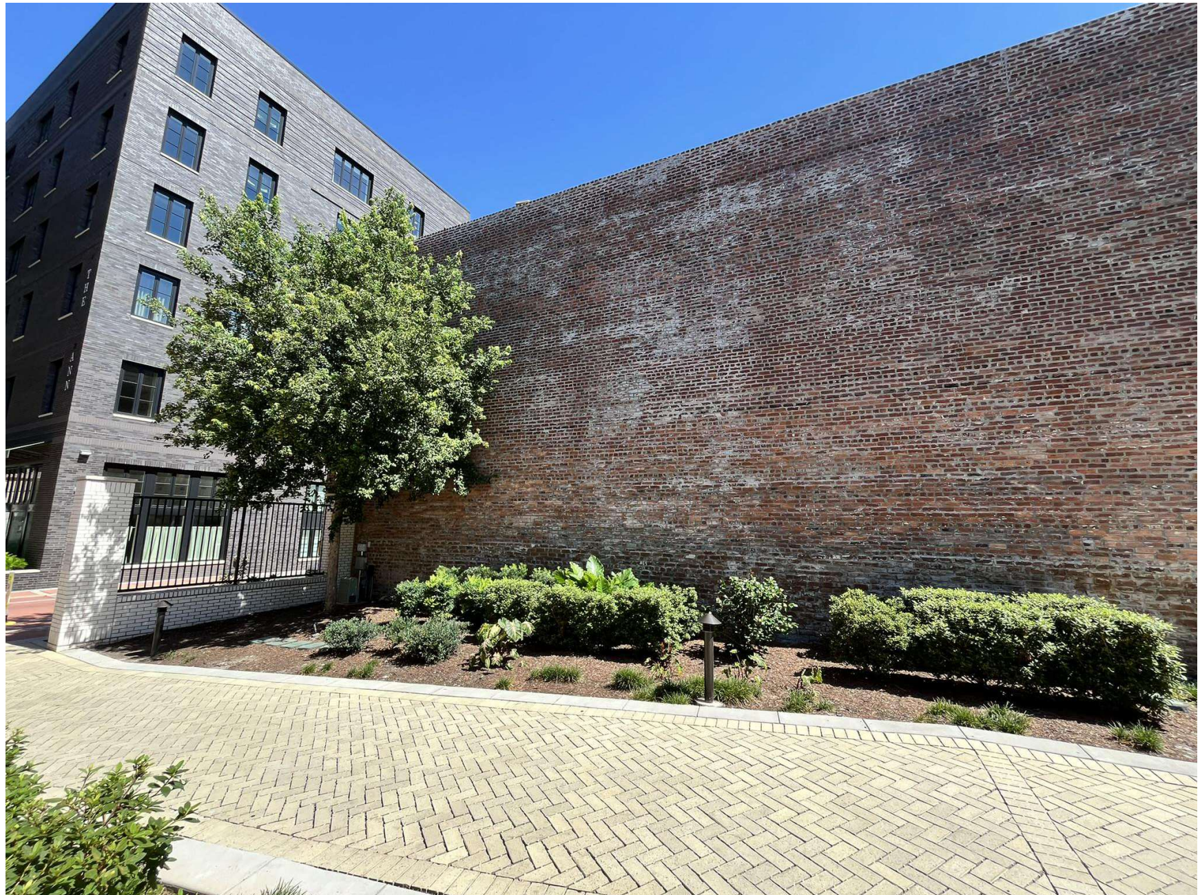
SOUTH COURTYARD FACADE
