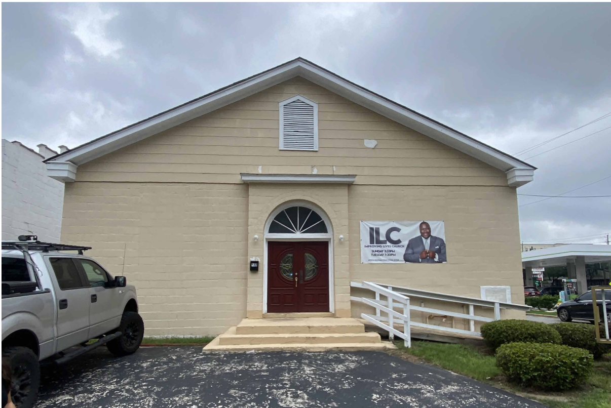
SOUTH FACADE, FROM BERRIEN ST.
