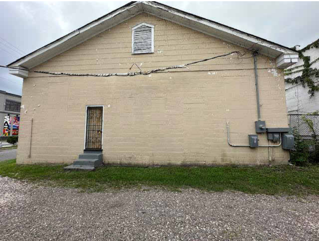
NORTH FACADE, FROM LANE
