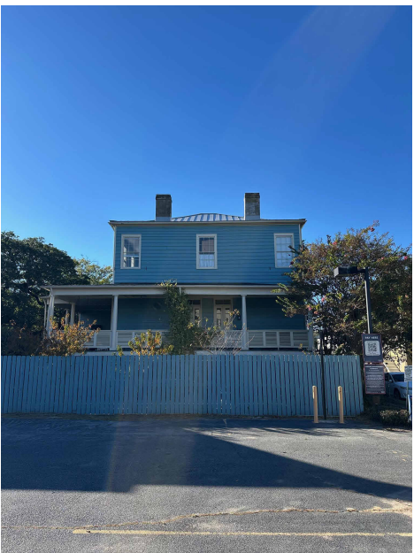
401 E. BROUGHTON ST - looking west
