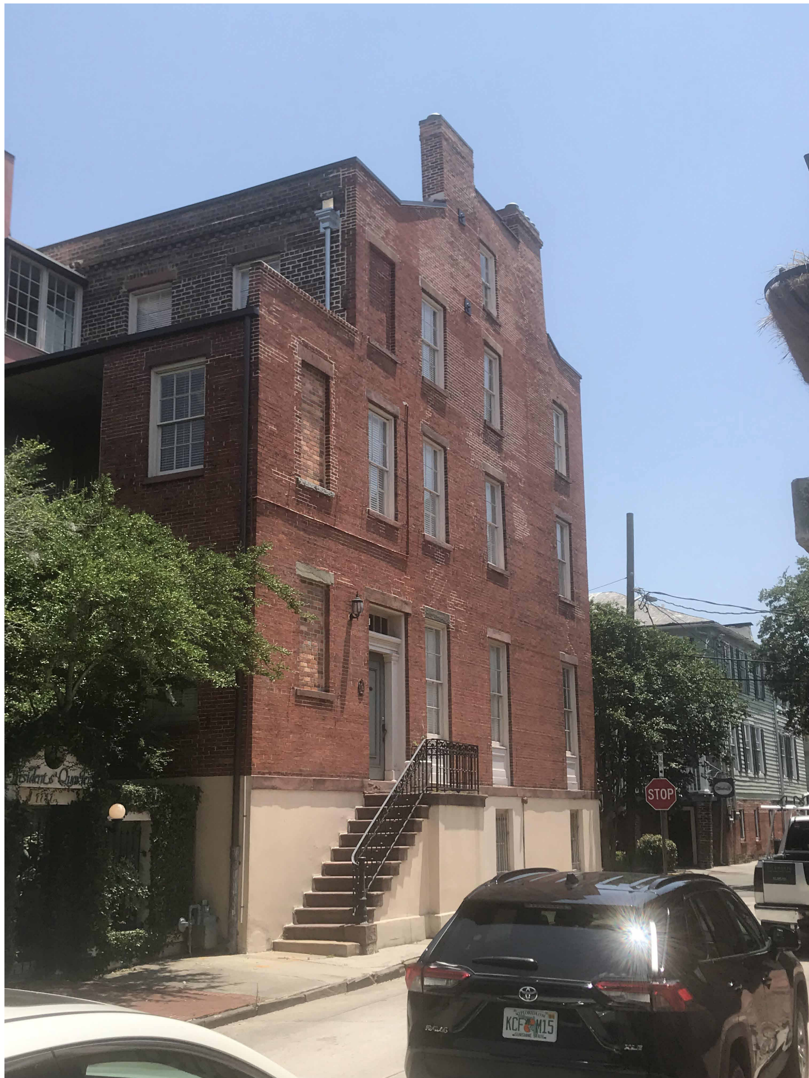
PHOTOS OF STAIR PRE - COLLAPSE
