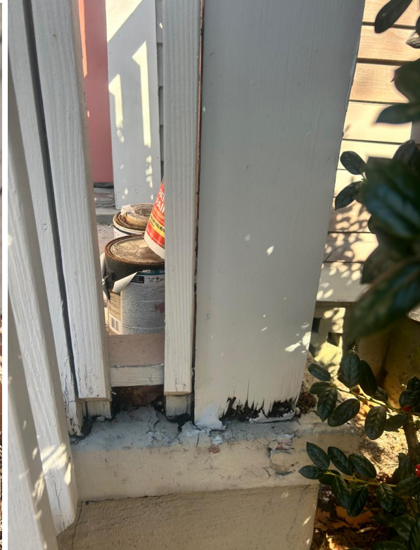
Unit 314 rotten step post handrail
