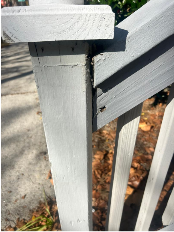
Unit 314 rotten step post handrail
