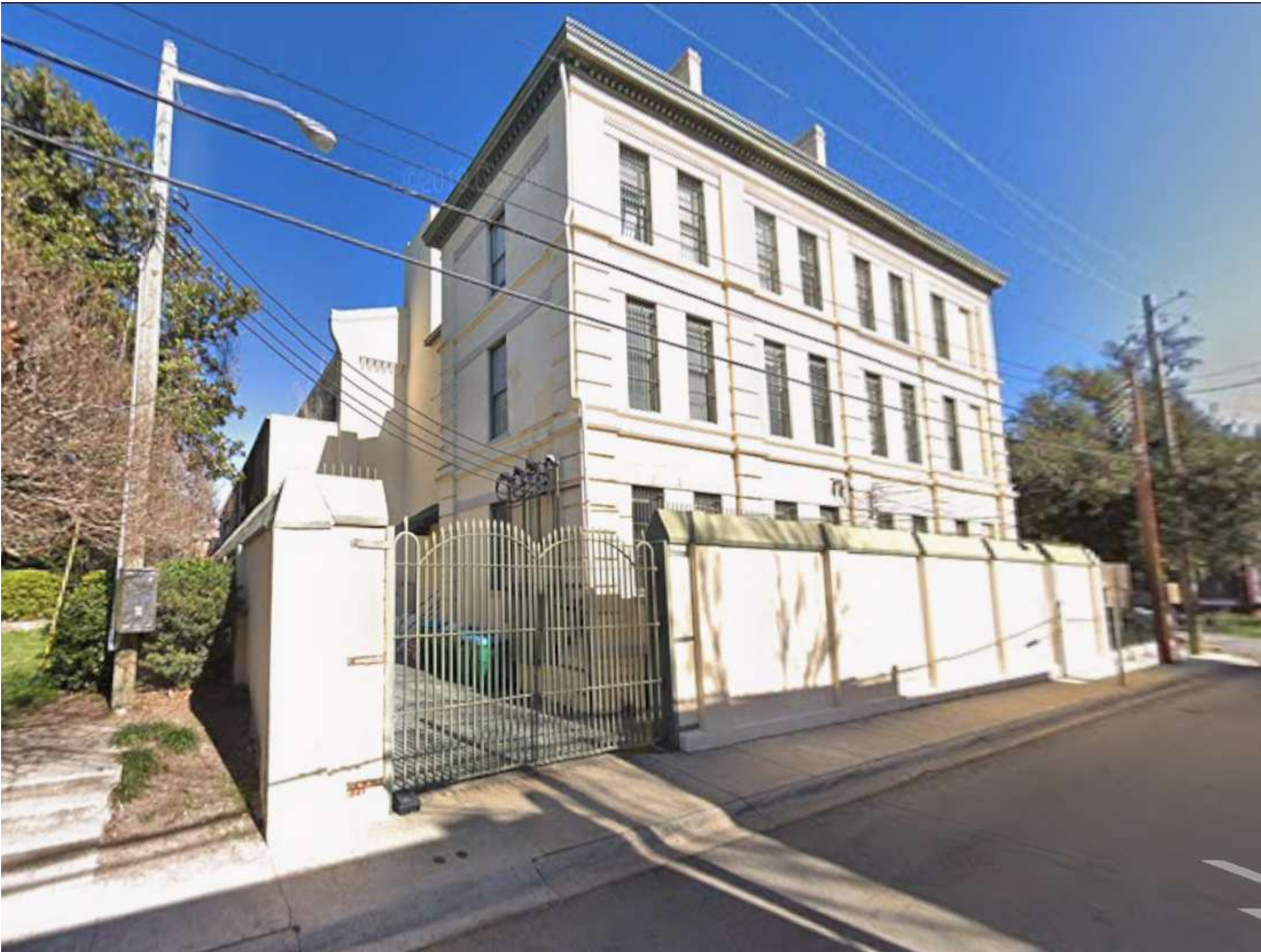
EAST PERRY LANE - LOOKING NORTHEAST
