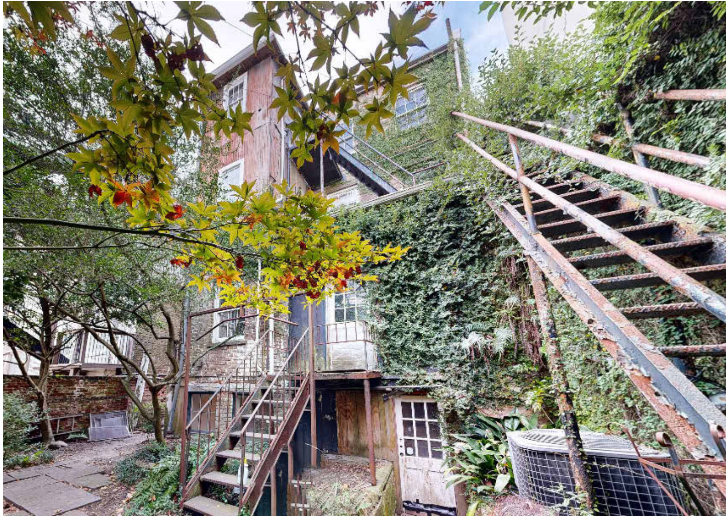
SOUTH FACADE FROM COURTYARD.
