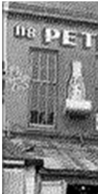
SIX-OVER-NINE DOUBLE- HUNG SASH WINDOW
