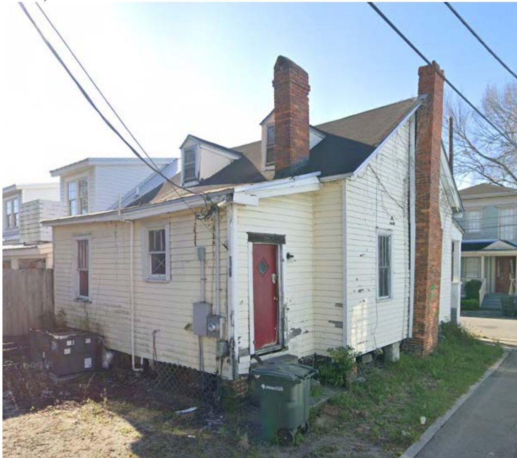
7. Photo showing the unoriginal exterior chimney and the interior chimney, most likely original
