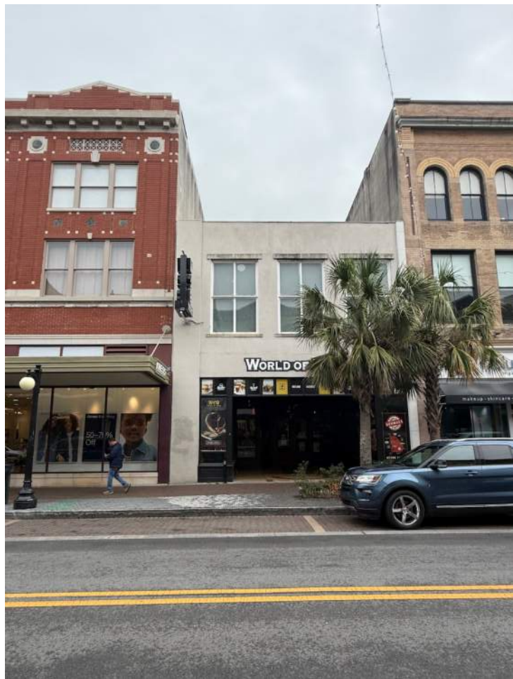
STOREFRONT FACADE FROM SOUTH SIDE OF W. BROUGHTON ST
