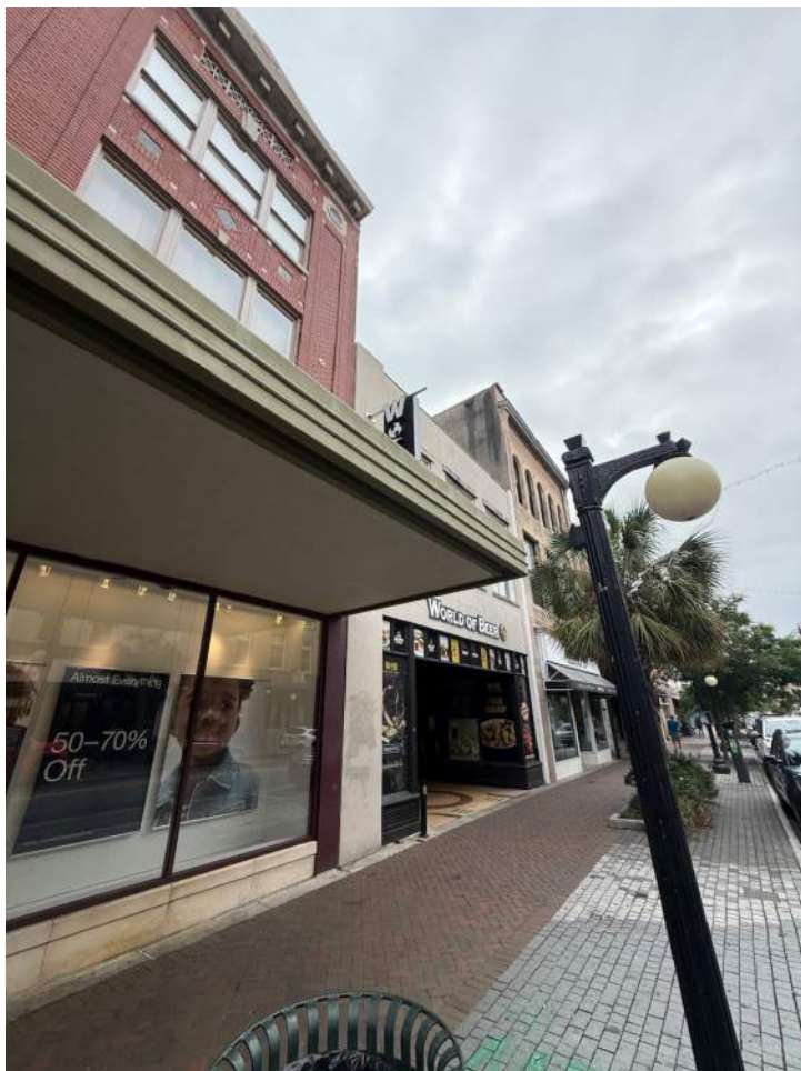
FACADE FROM WEST APPROACH ALONG W. BROUGHTON ST
