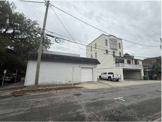
E HULL STREET LOOKING TOWARDS 225 HOUSTON STREET
