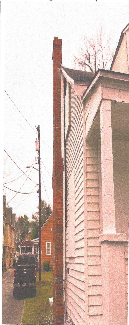
Prior to Removal
