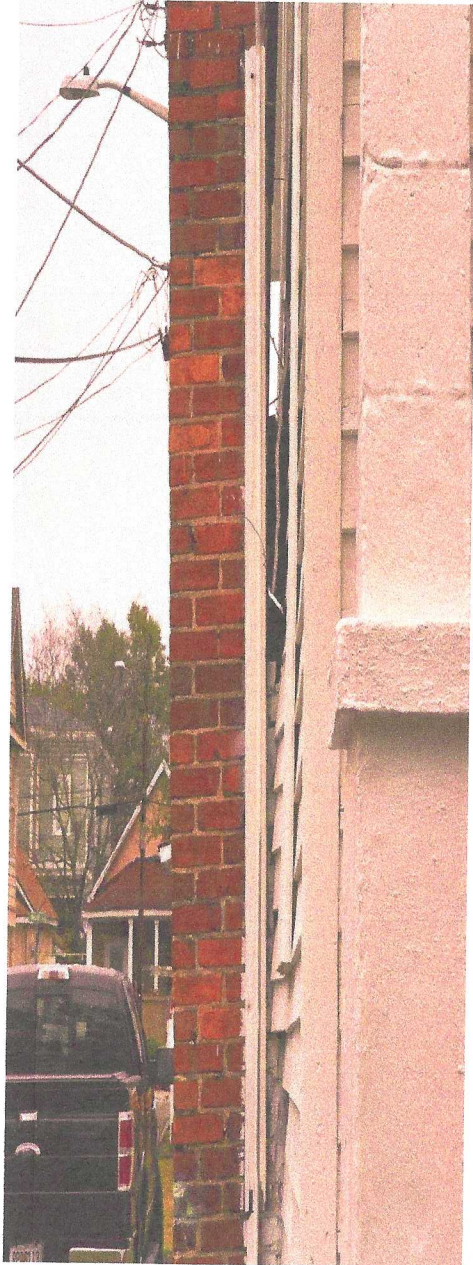
Prior to Removal
