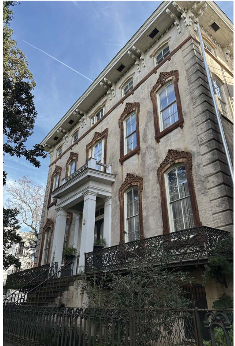
View from West Gordon Street
