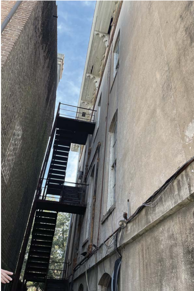
View of West Elevation from West Gordon Lane side.
