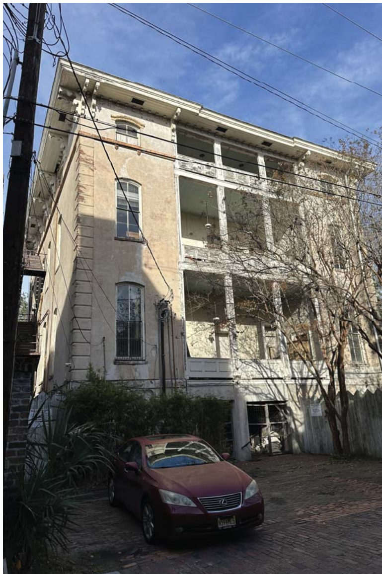
View of South Elevation from West Gordon Lane
