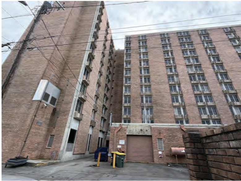
Existing Building Across the Lane
