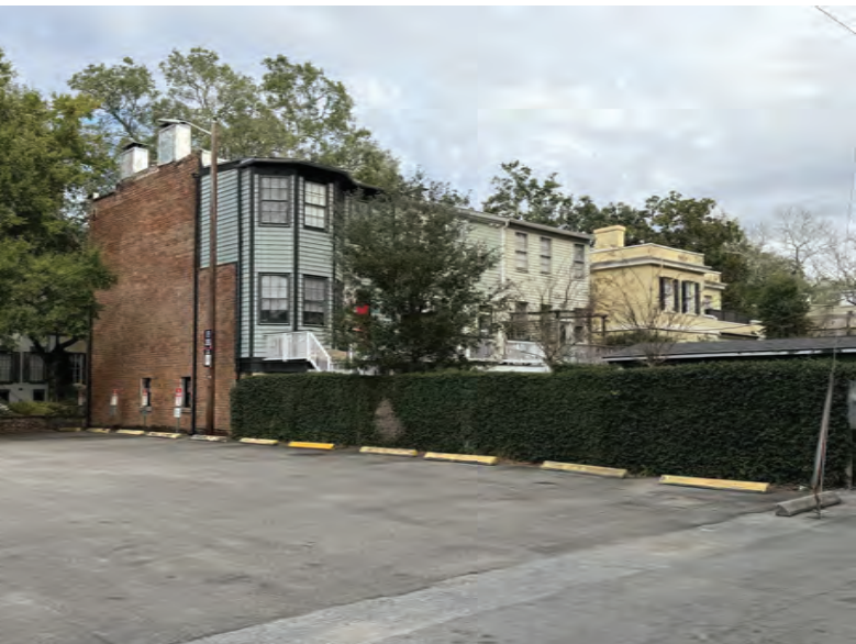
Back SW View of Townhomes
