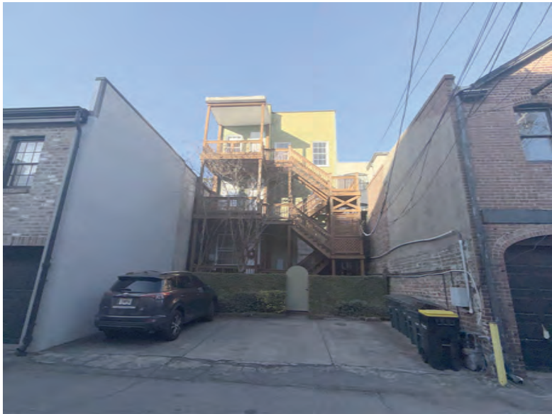
E. Jones Lane * Back Addition and Porch
