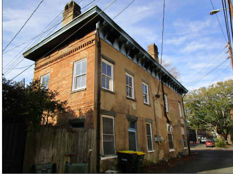
REAR & W. GORDON LANE ELEVATIONS (BLUE CORNICE SECTION OF BUILDING)
