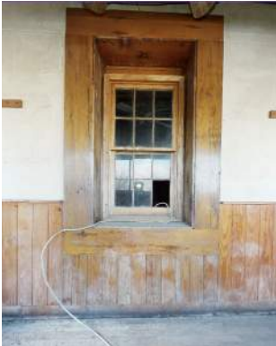
EXISTING INTERIOR WINDOWS
