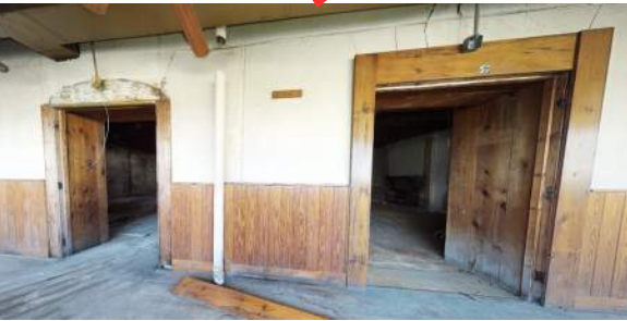
EXISTING INTERIOR OPENINGS
