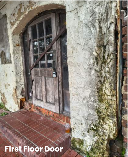
Typical Condition of existing Stucco
