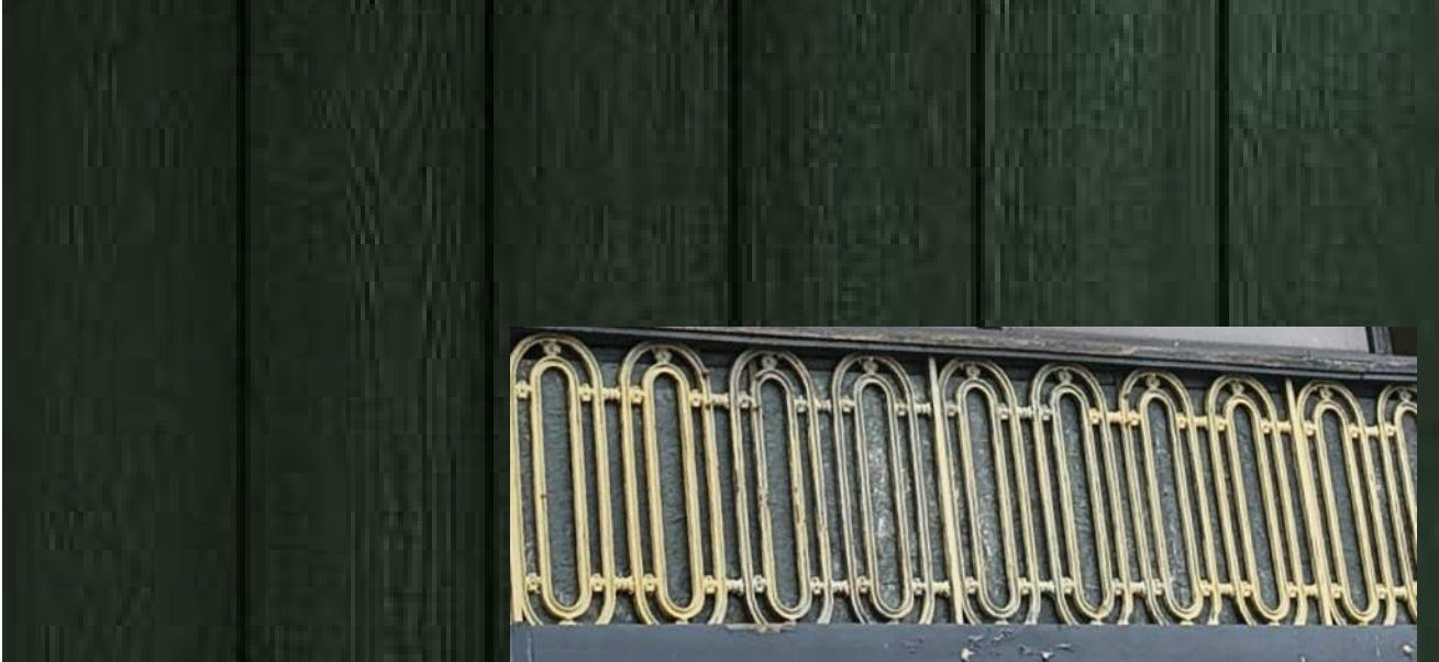
Balcony Siding – Hardipanel Vertical Siding Painted Sherwin Williams Greenblack SW 6994 Restored Decorative Metal Trim
