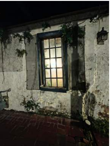
EXISTING EXTERIOR WINDOWS
