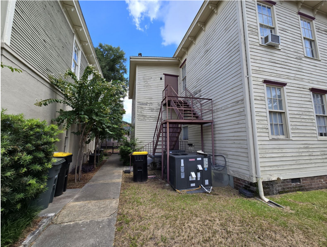
Photo 5 – North side / pedestrian easement between building and 434 Jefferson St
