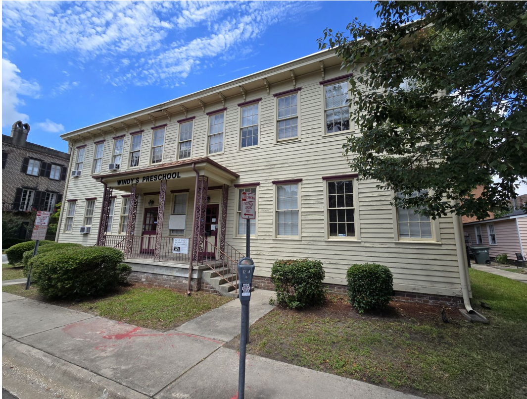
Photo 1 – East (Tattnall Street) front elevation
