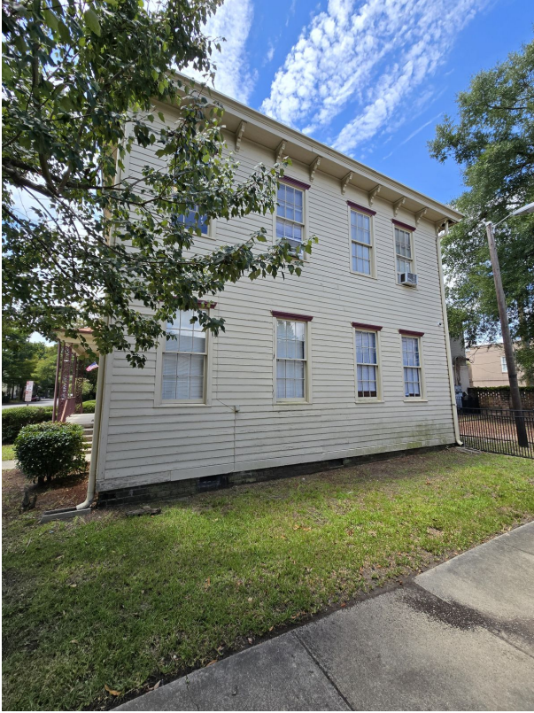
Photo 3 – South elevation along W. Wayne Street
