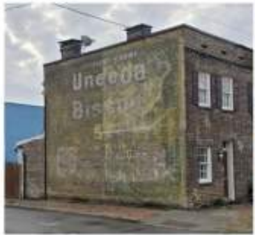
Current State Condition
