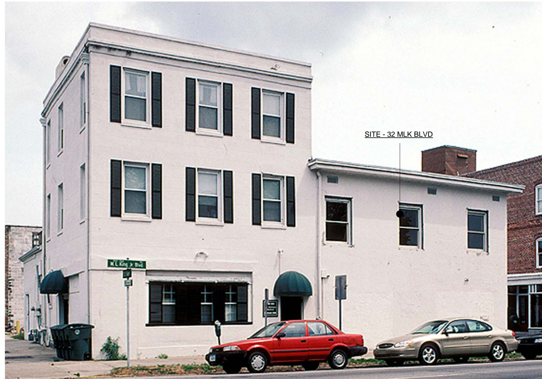
32 MLK BLVD. - 2001 A LATER PHOTOGRAPH, TAKEN IN 2001 ONE, INDICATES THE MLK BLVD. STOREFRONT WAS INFILLED, WHILE THREE WINDOW OPENINGS WERE ADDED ON THE SECOND FLOOR REVIEWING THE WIDER, TRUNCATED PROPORTION OF THE SECOND FLOOR WINDOWS, IT IS SAFE TO ASSUME, THEY ARE NOT HISTORIC. ADDITIONALLY, FROM THE INTERIOR OF THE BUILDING, THE CENTER BEAM OF THE SECOND FLOOR FALLS AT THE HEADER OF THE CENTER WINDOW WHICH WOULD NOT BE AN APPROPRIATE/HISTORIC METHOD OF CONSTRUCTION. (IMAGE D - SHEET A4). ADDITIONALLY, THIS BEAM AT THE HEADER CONTRIBUTES TO THE BUILDINGS STRUCTURAL DEFICIENCIES, NOTED IN THE STRUCTURAL REPORT, ITEM 3 - PAGE 2 OF 14.
