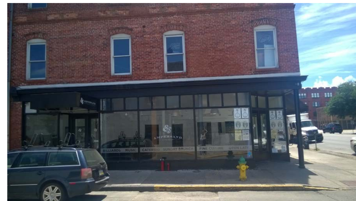
IMAGE D: STOREFRONT OF 3 STORY BUILDING, SOUTH OF CONGRESS FROM SITE
