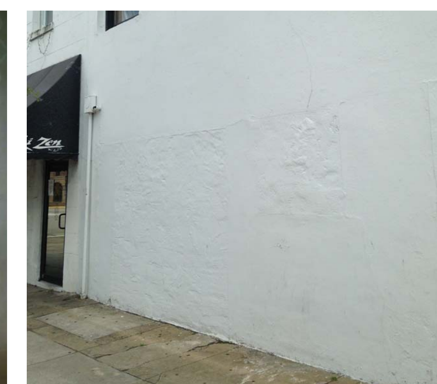
L. FIRST FLOOR, INFILLED OPENINGS VISIBLE ALONG MLK JR. BLVD EXTERIOR
