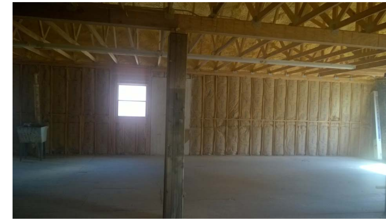
C. SECOND FLOOR, NEW CONSTRUCTION ENTIRE SOUTH WALL & ROOF STRUCTURE
