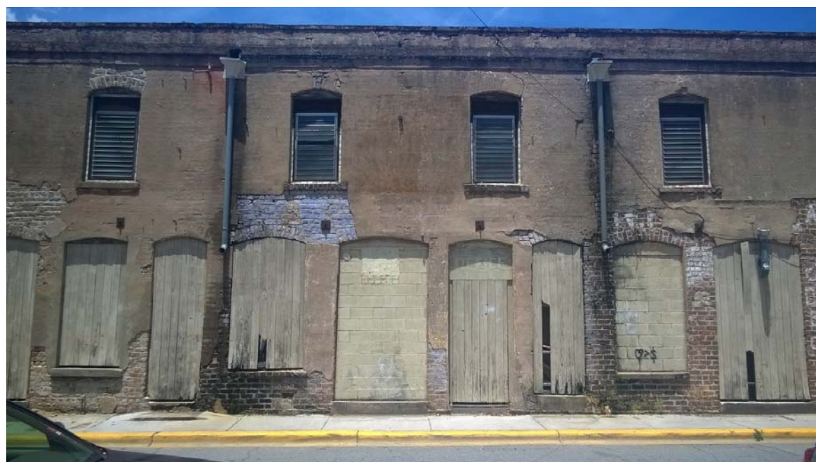
IMAGE F: VACANT, 2 STORY STRUCTURE, SECOND PARCEL EAST OF SITE
