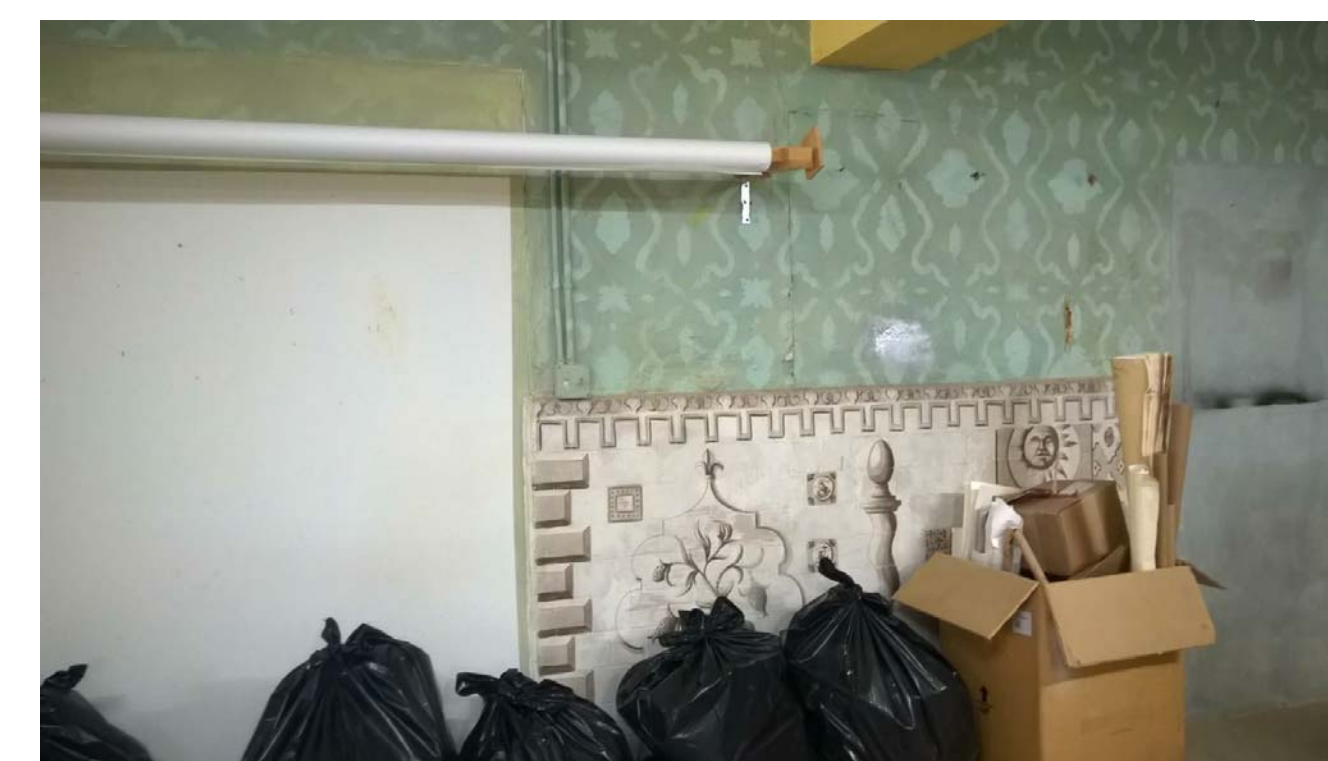
K. FIRST FLOOR, VIEW SOUTHWEST, INFILLED OPENINGS VISIBLE ALONG MLK JR. BLVD
