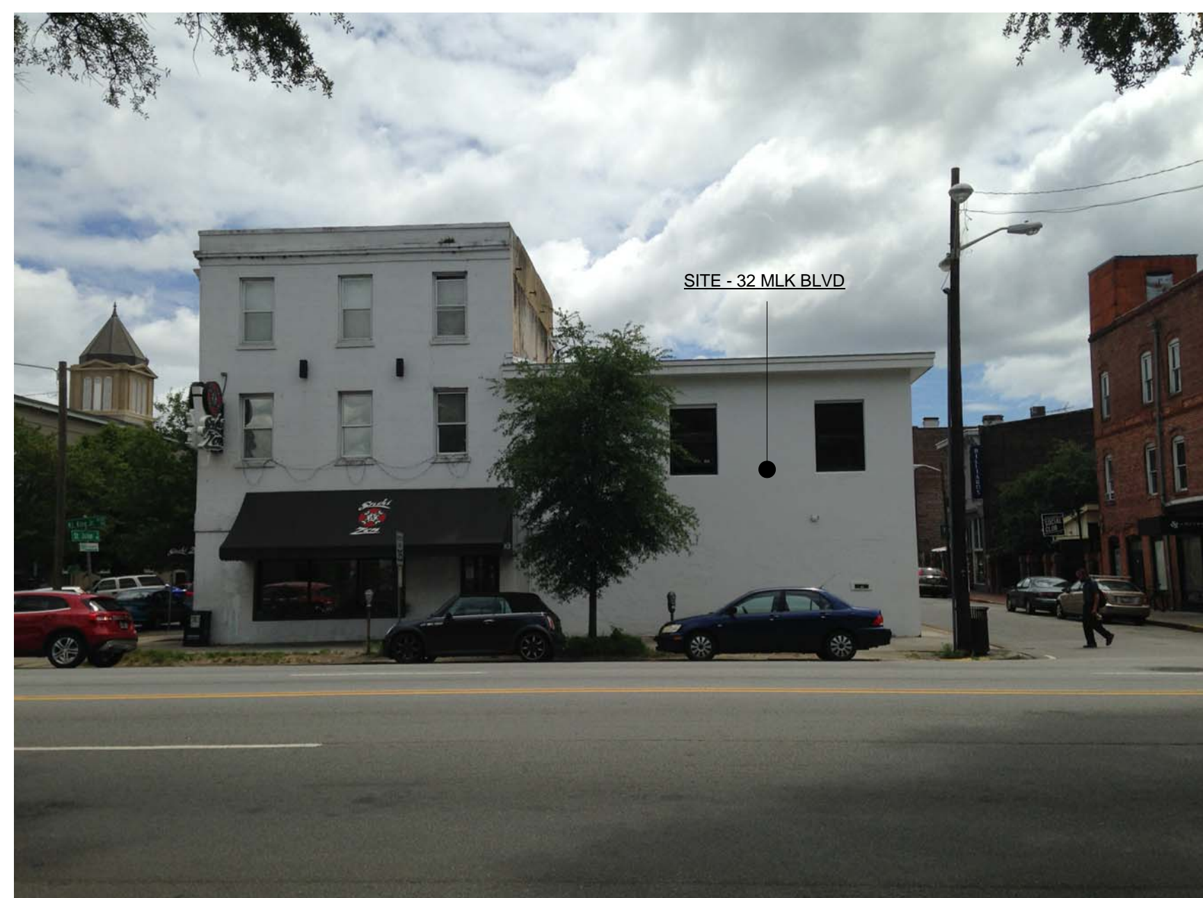
32 MLK BLVD - CURRENT 2015 TODAY, WHEN REVIEWING THE WEST FACADE OF 32 MLK BLVD, IT APPEARS TO HAVE CHANGED MINIMALLY SINCE THE 2001 PHOTOGRAPH. HOWEVER, REVIEWING THE WEST FACADE FROM THE INTERIOR, SIGNIFICANT MODIFICATIONS ARE VISIBLE, APPROXIMATELY TWO YEARS AGO, THE PREVIOUS OWNER REPAIRED THE ROOF TO THE EXTENT OF COMPLETE ROOF REMOVAL, REPLACING THE HISTORIC ROOF WITH PRE-ENGINEERED ROOF TRUSSES. (IMAGES A-E - SHEET A4) IN ADDITION TO COMPLETE REPLACEMENT OF THE ROOF, THE ENTIRE SOUTH WALL WAS RERAMMED FROM THE FIRST FLOOR UP, VISIBLE IN IMAGES B-C, SHEET A4. THE MULTIPLE MODIFICATIONS TO THIS BUILDING, SPECIFICALLY THE LOSS OF THE THIRD FLOOR LEFT A BUILDING THAT NOT ONLY LACKS HISTORICAL PROPORTIONS AND SCALE OF SURROUNDING CONTEXT, BUT ALSO HAS MULTIPLE STRUCTURAL DEFICIENCIES. IN ORDER TO STABILIZE AND REVONATE THE BUILDING TO MEET STRUCTURAL CODE REQUIREMENTS, THE COST WOULD EXCEED THE PURCHASE PRICE OF THE PROPERTY BY NEARLY DOUBLE.
