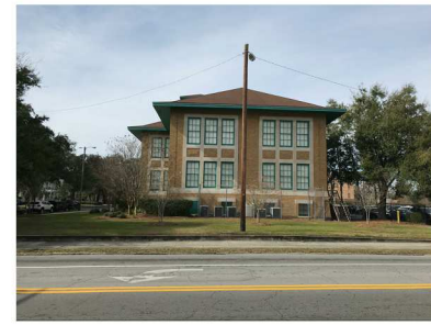
SCAD'S WALLIN HALL (SIDE FACADE ALONG HABERSHAM ST.)
